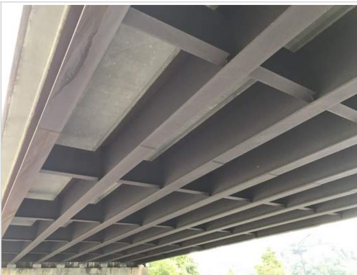
Soffit & superstructure facing abutment 1
