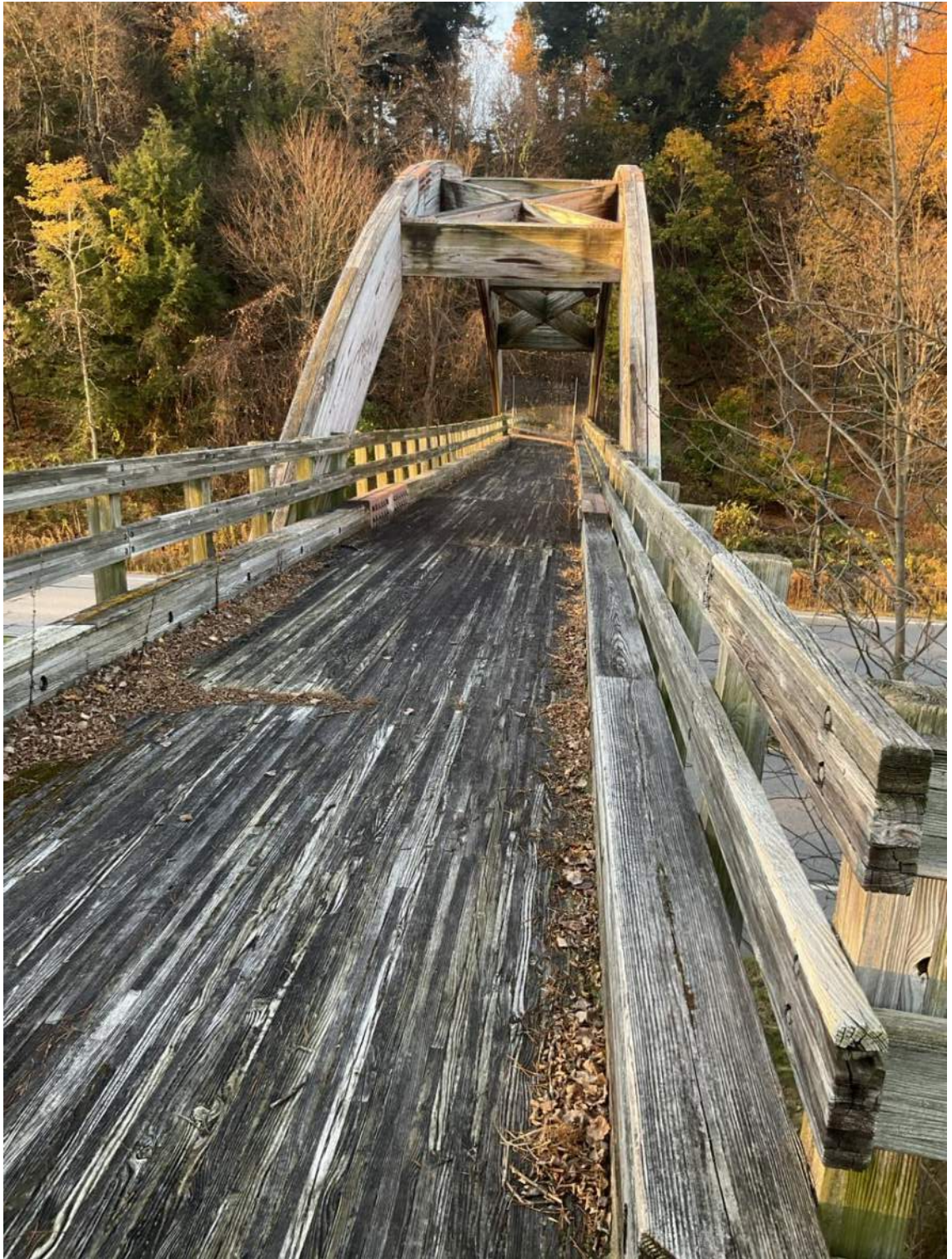
Photo 1 Facing west on the "Bridge to Nowhere" over VT 127.
