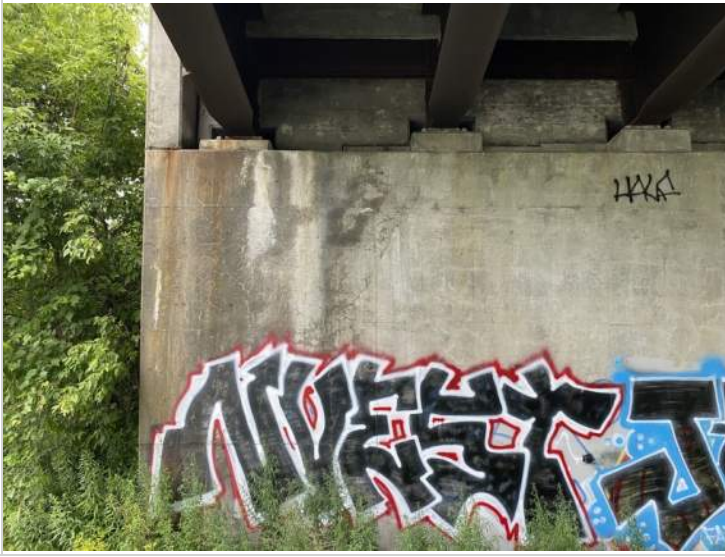
Abutment #2 Northern End
