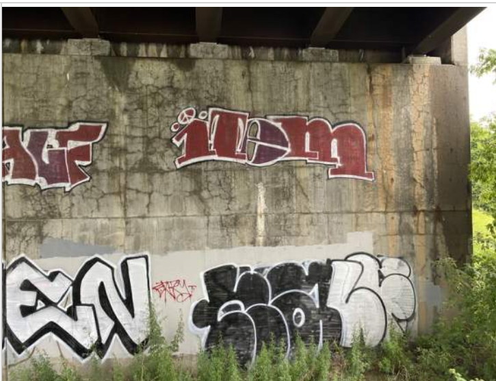
Northern End of Abutment #1
