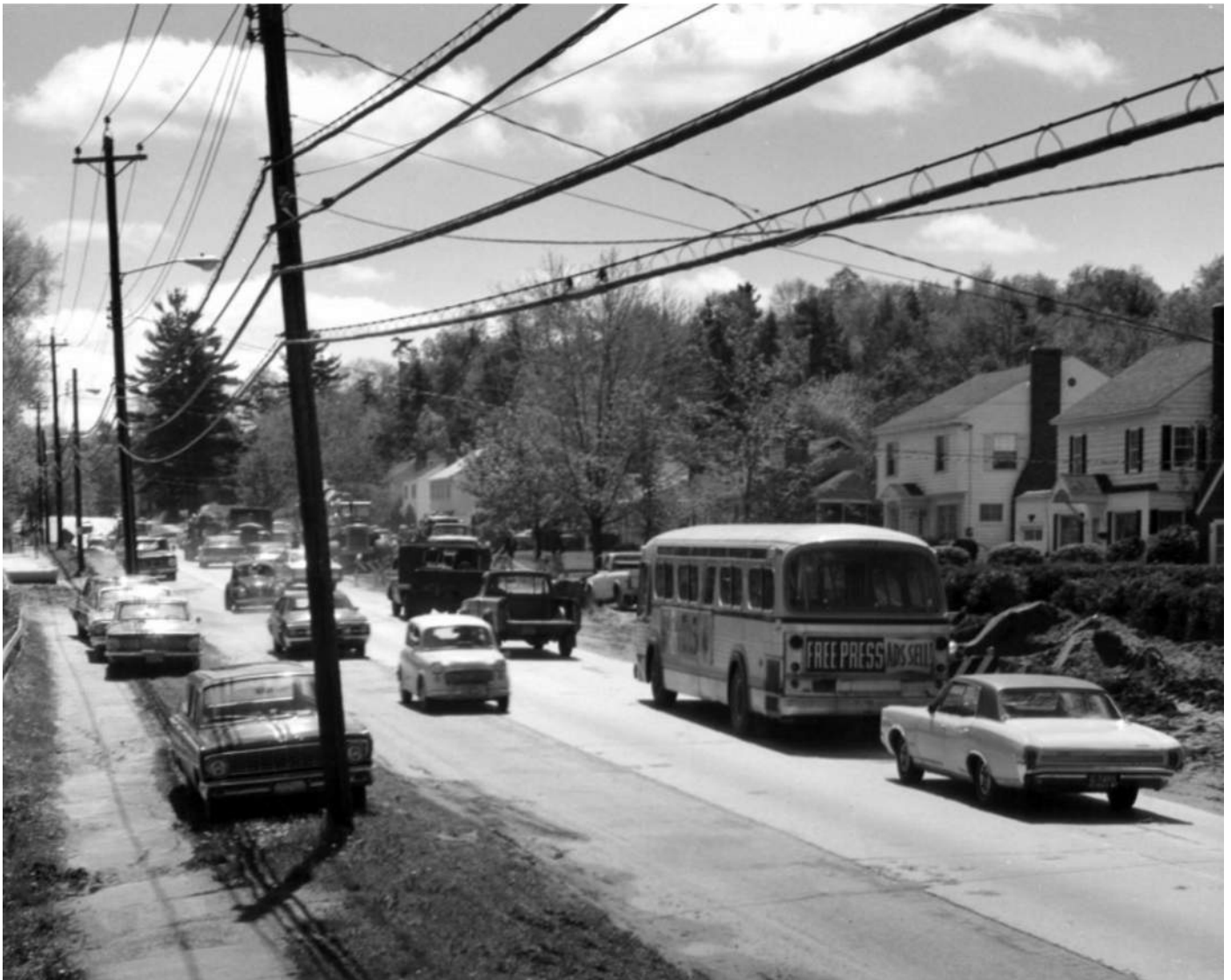
Figure 9: North Avenue, looking south. The houses at right at 821 and 815 North Avenue. The image is dated 1969, and the construction scene shows the widening of North Avenue as part of the VT 127 interchange. Source: UVM Landscape Change file LS08803_000.
