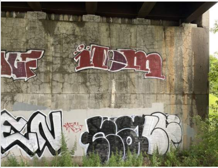
Northern End of Abutment #1
