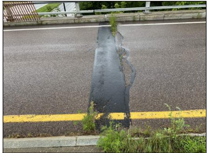
Asphaltic Plug Joint on South Side of Abutment #1
