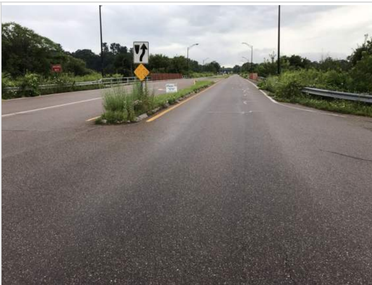
Abutment 2 approach (East)
