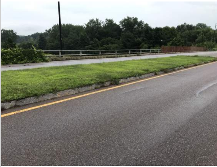
North bridge rail
