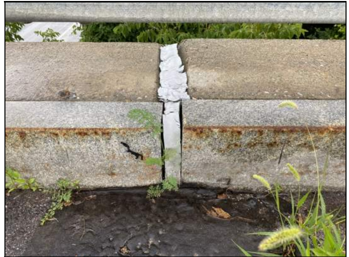
Curb Seal (Southern End of Abutment #1)
