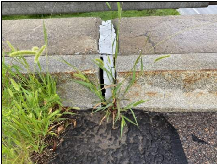
Curb Seal (Northern End of Abutment #1)
