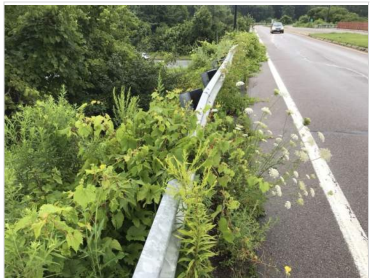
North approach rail to abutment 1
