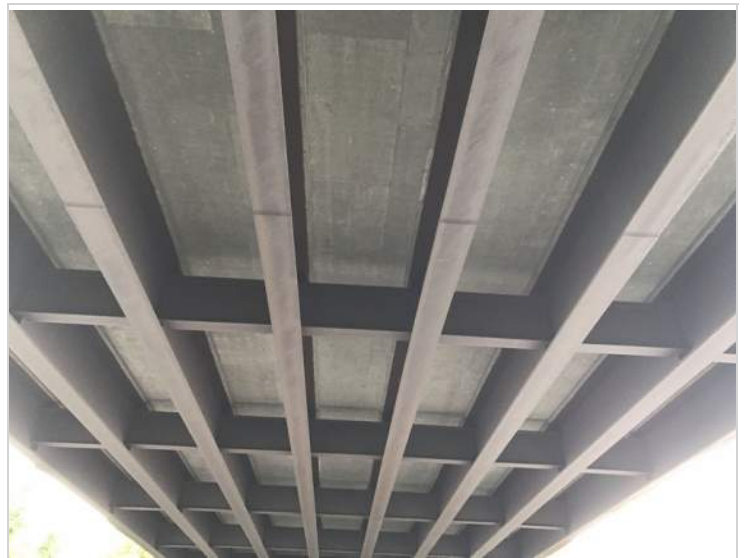
Soffit & superstructure facing abutment 2
