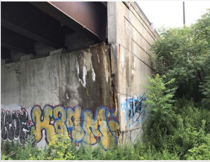
South end of abutment 2 at wingwall 4
