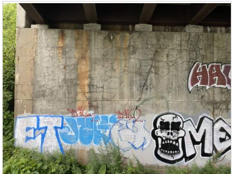
Southern End of Abutment #1
