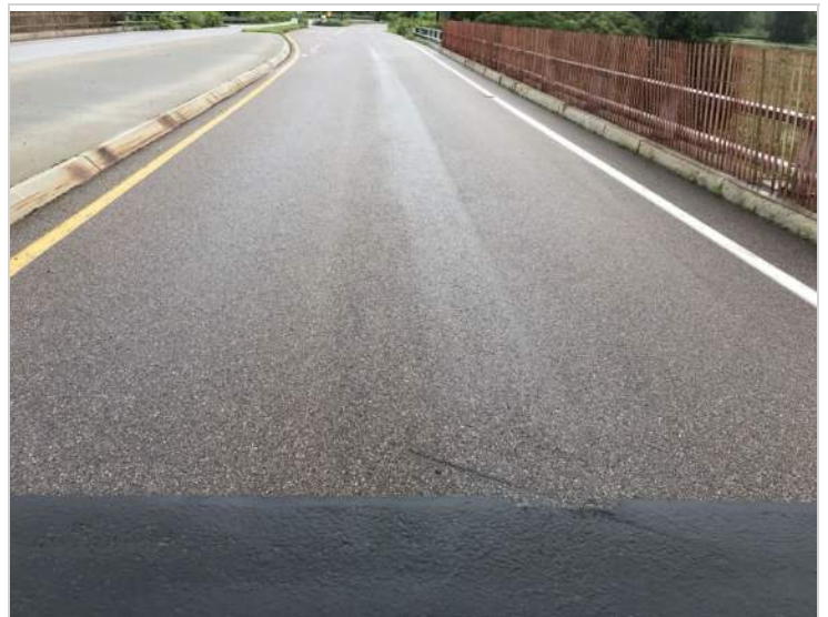
Wearing surface Eastbound lane from abutment 1
