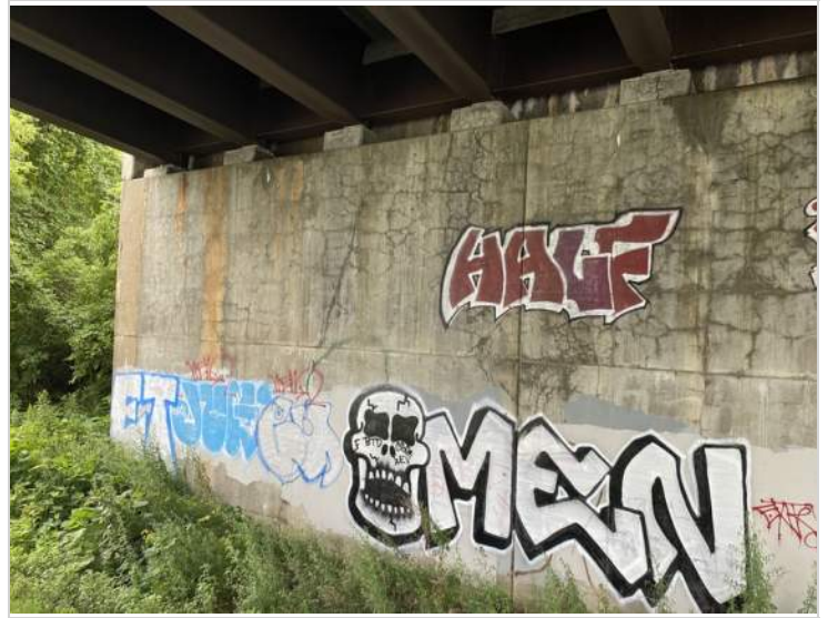
Southern End of Abutment #1
