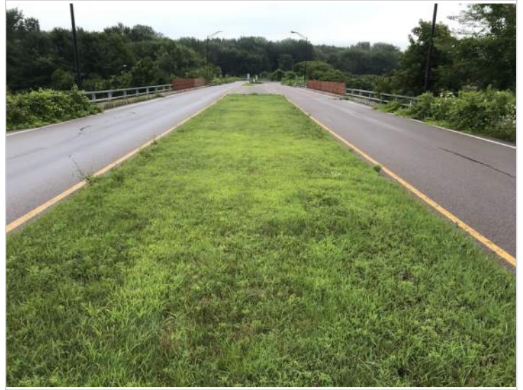
Abutment 1 approach (West)
