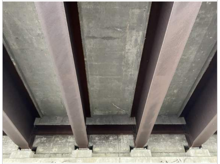
Bay #4 at Abutment #2
