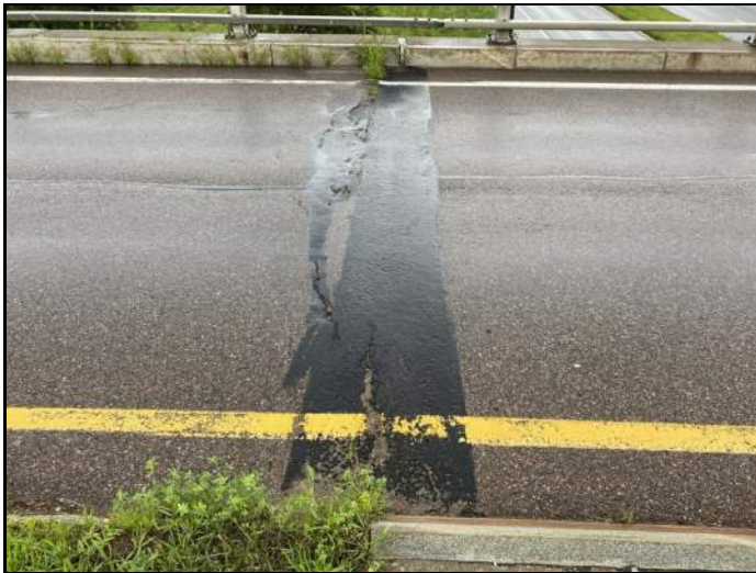
Asphaltic Plug Joint on North Side of Abutment #1
