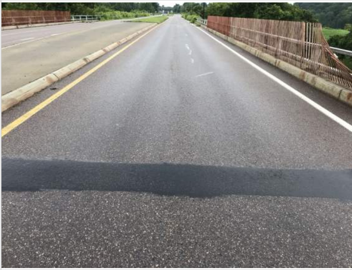
Wearing surface Westbound lane from abutment 2
