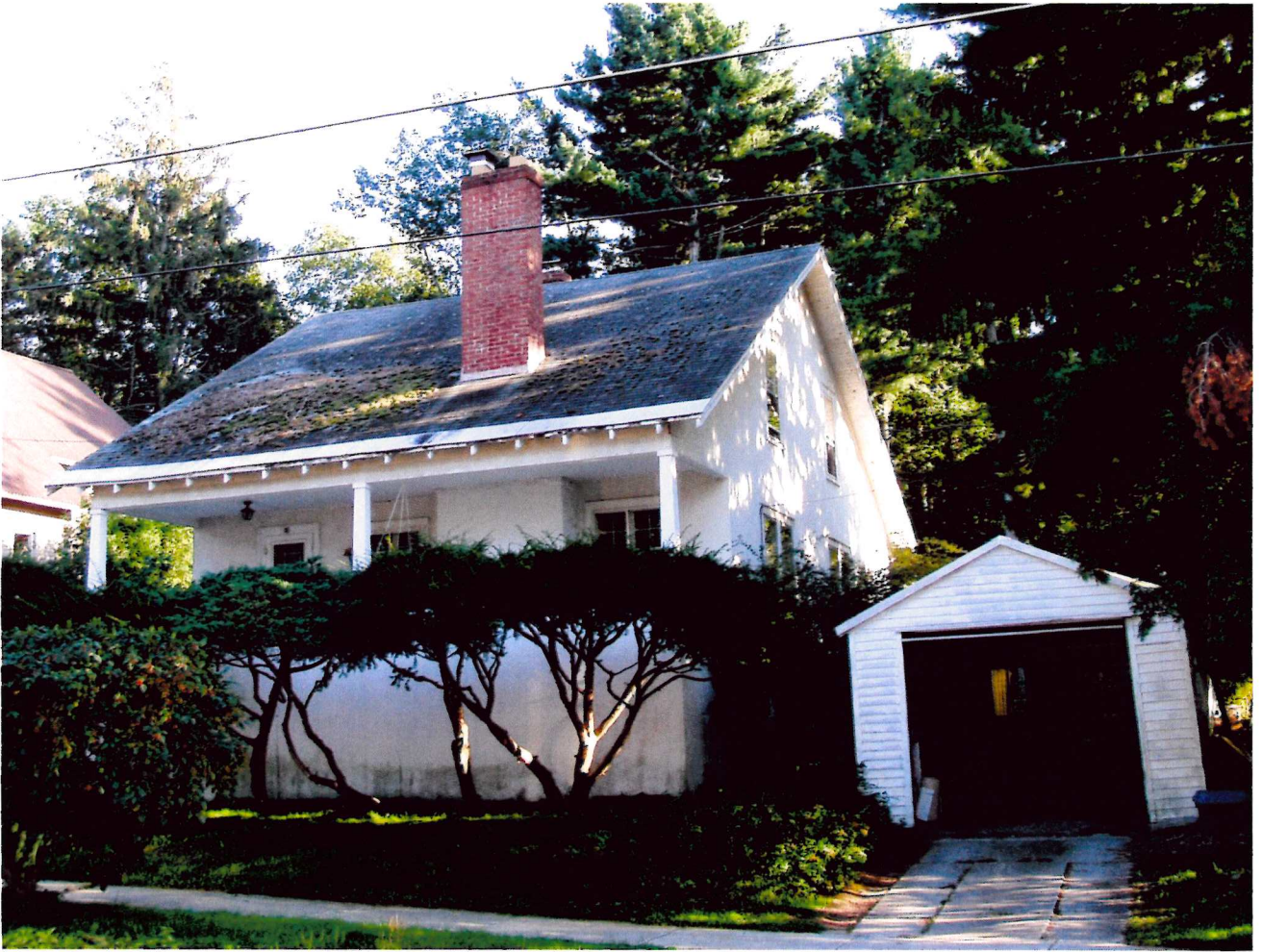
VERMONT DIV. FOR HISTORIC PRESERVATION Property Name: 49 henderson terrace Survey #: Direction of View: Filename: 49 henderson terrace.JPG Photographer:
