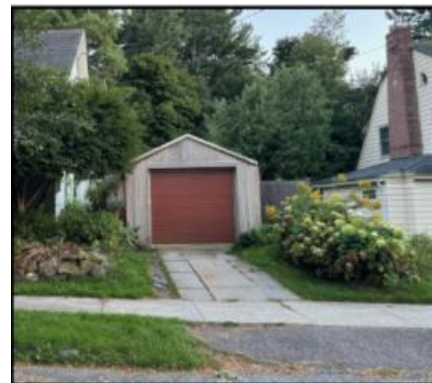
EXISTING FRONT VIEW
