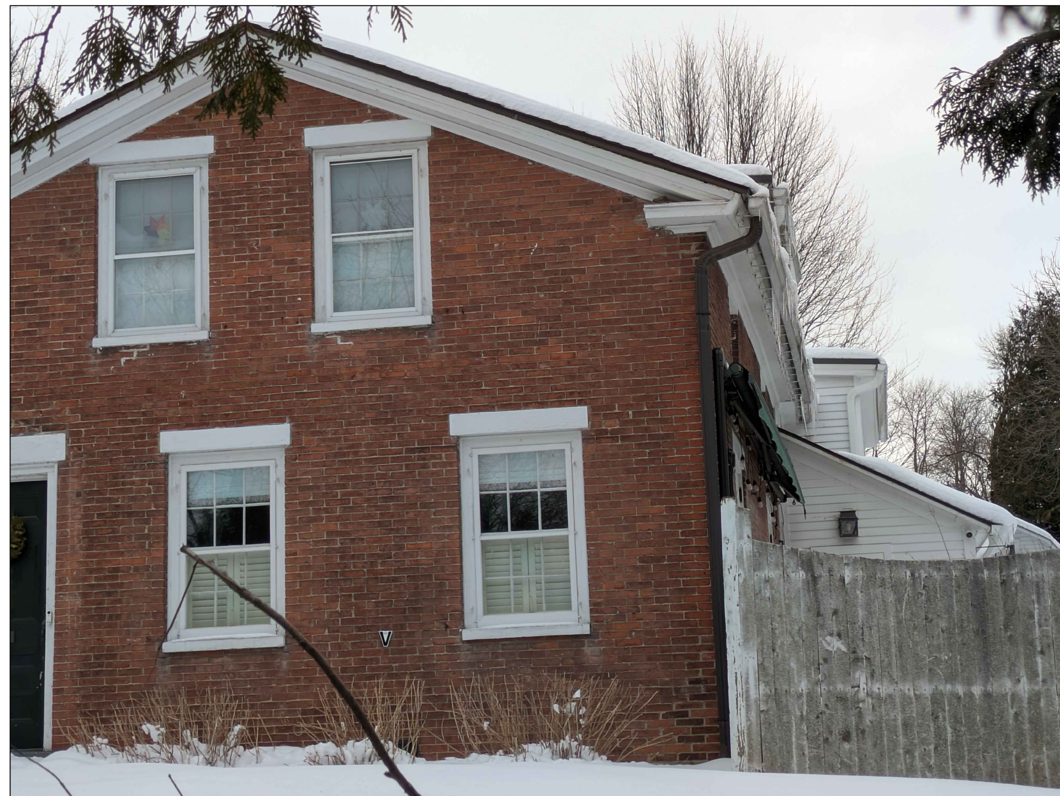
North West Corner
