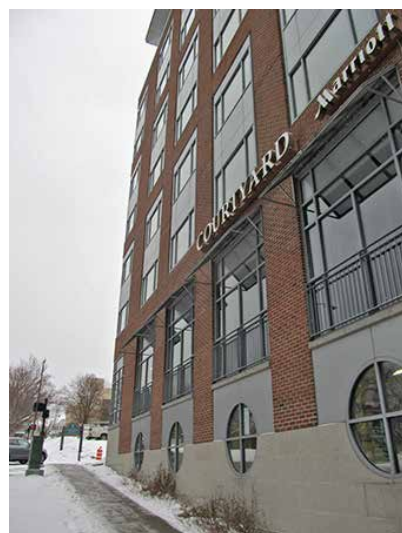
EXISTING SIGN TO BE REMOVED
