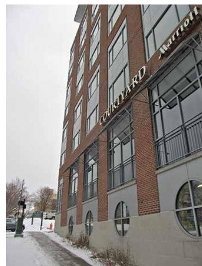
EXISTING SIGN TO BE REMOVED
