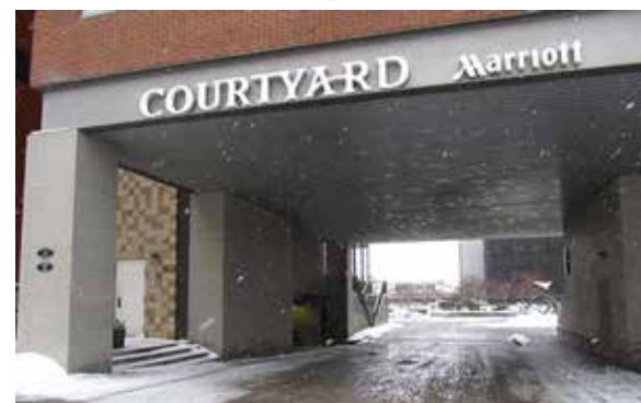
EXISTING SIGN TO BE REMOVED
