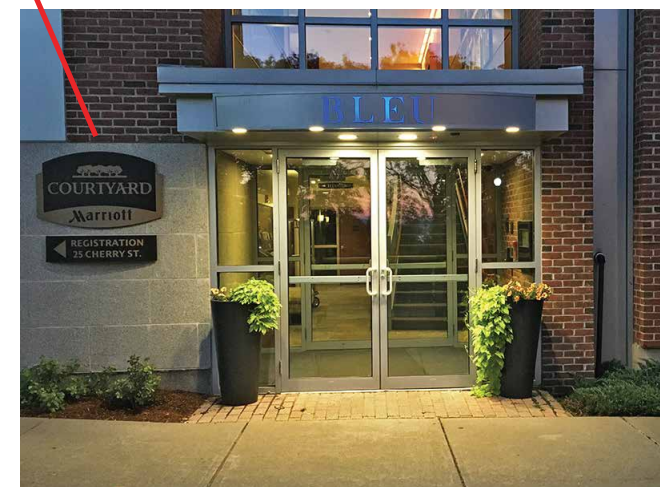
EXISTING SIGNS TO BE REMOVED
