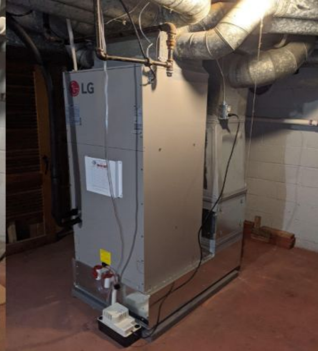
Heatpump Heat Exchanger
