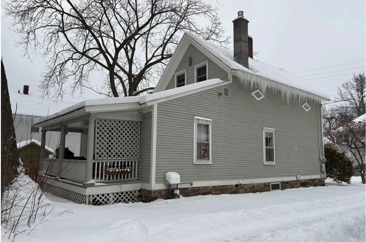
Rear/Side of home viewed from Hayward St. - Northeast Facing
