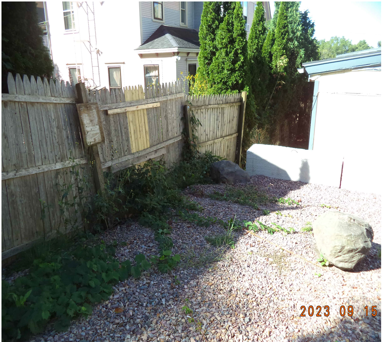
Photograph 1 – View of boundary fence (250 S. Union Side), looking southwest towards 254 S. Union Residence
