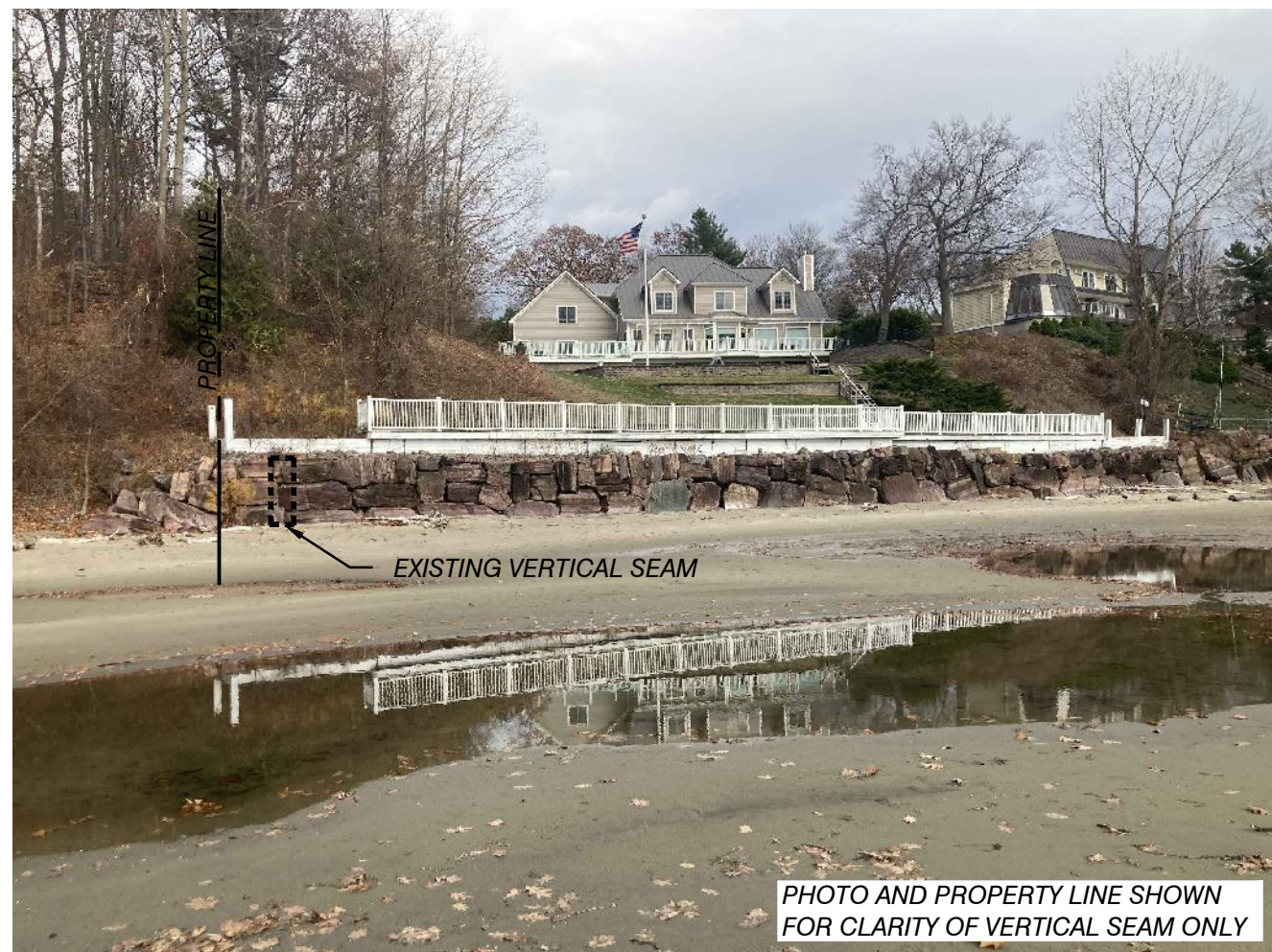
EXISTING WALL IMAGE
