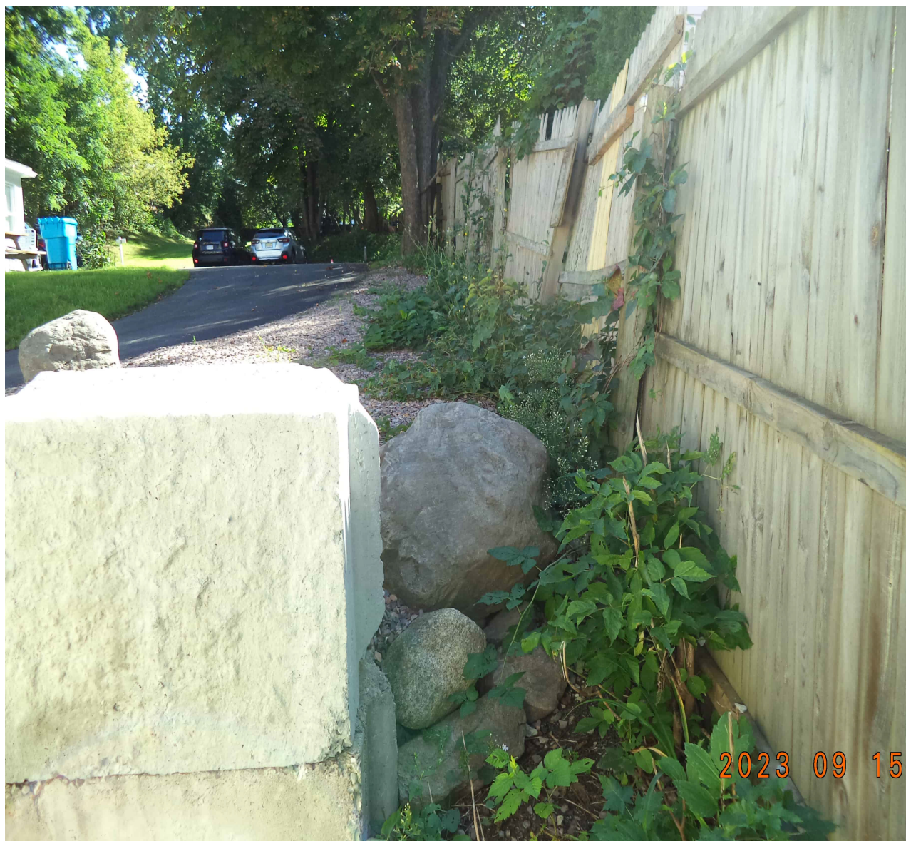
Photograph 3 - View of boundary fence (250 S Union Side), looking north.
