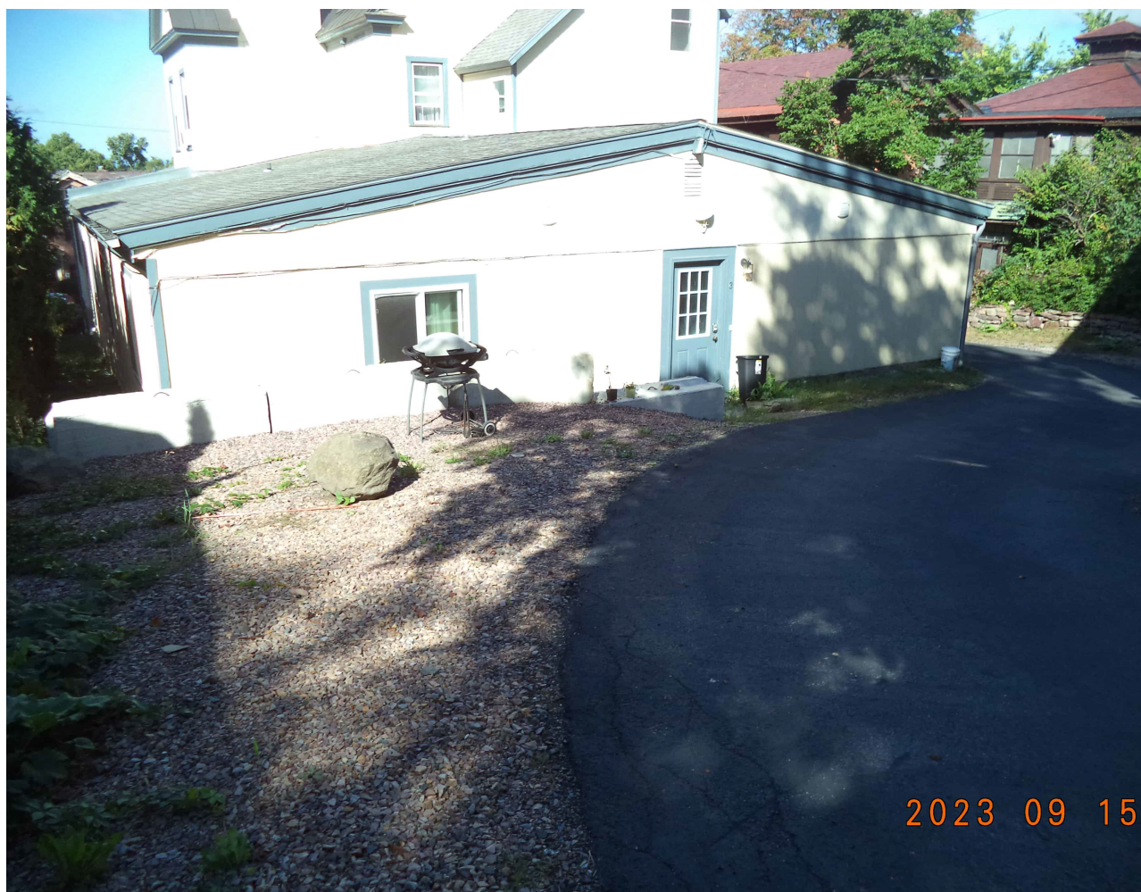
Photograph 5 - View of regraded driveway at 250 S Union Street, looking west
