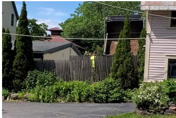
6. June 9, 2023. Workers offloading a 15-yard load of hard pack driveway material along the border.
