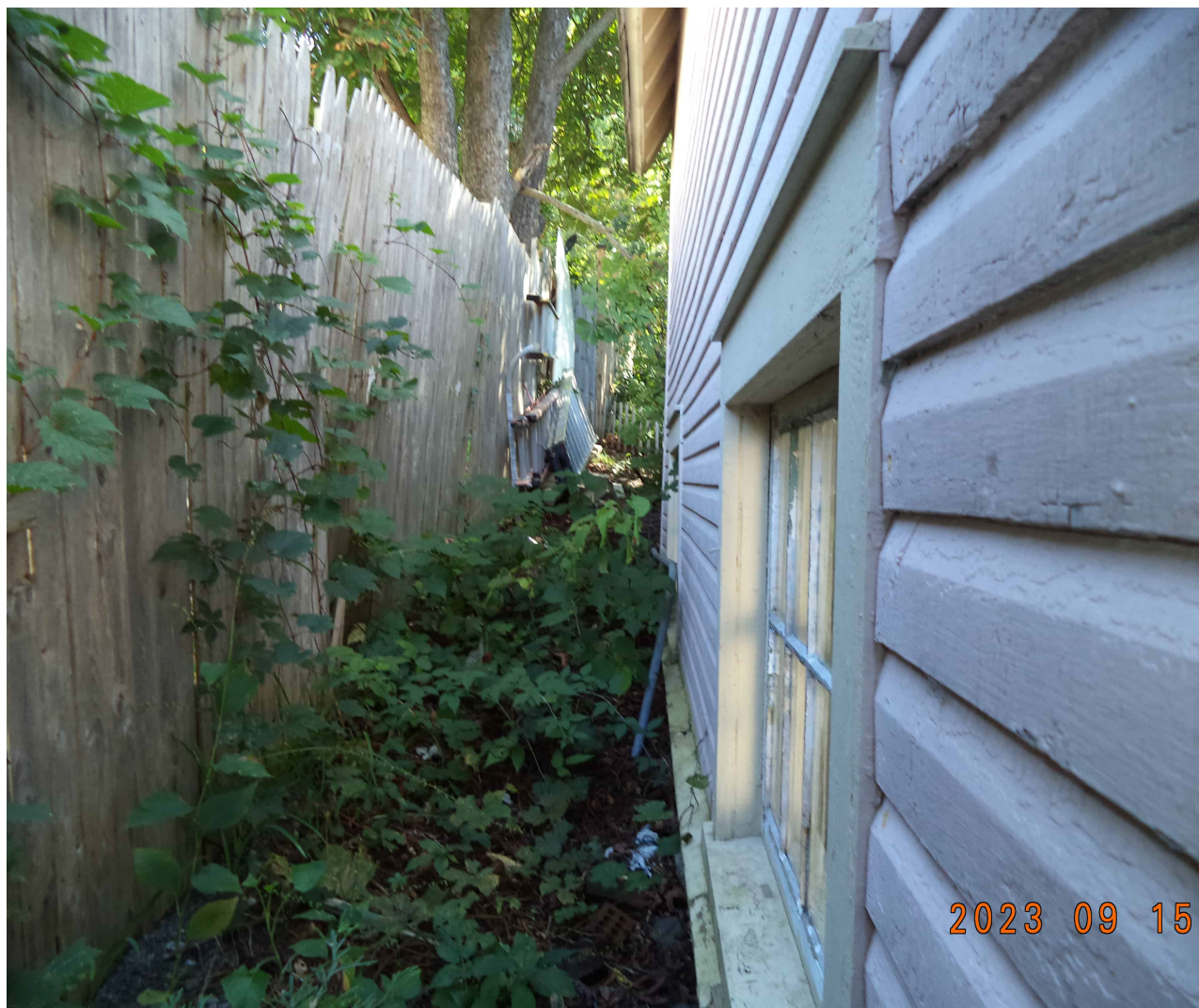
Photograph 4 - View of boundary fence (254 S Union Side), looking north.
