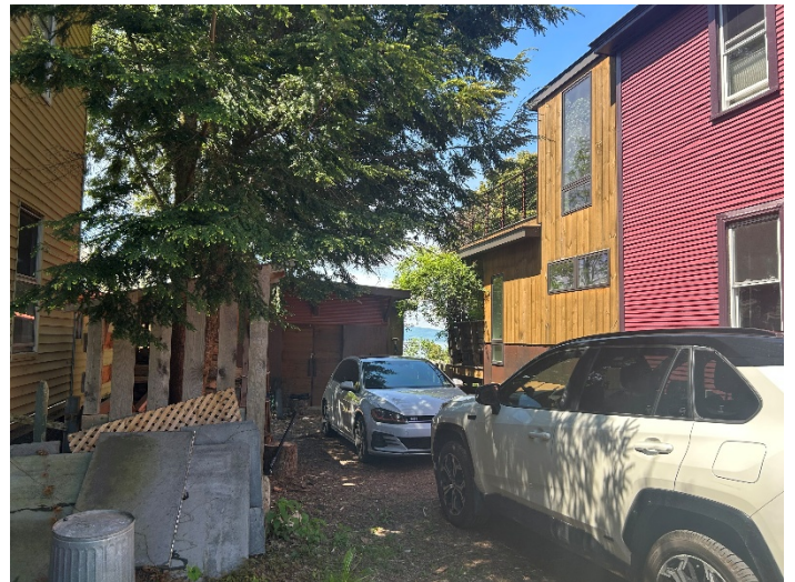
South side of existing house – looking at original house and previous addition plus ADU completed in 2015
