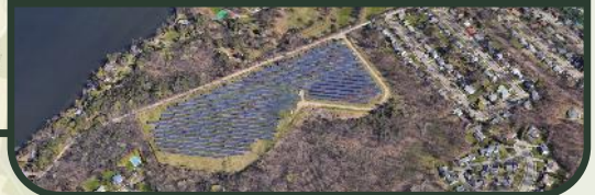
New North End Solar Array
