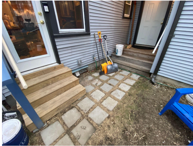
Photos of Existing Deck & Low grade Steps, Side Porch to Convert, Steps to move
