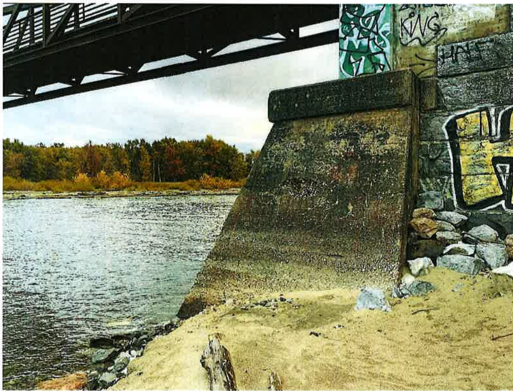
Southern Abutment – Downstream – Fill is small granular material covered in fine sand.
