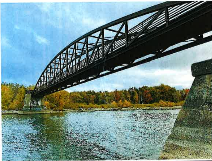
Bridge from southern abutment looking north.
