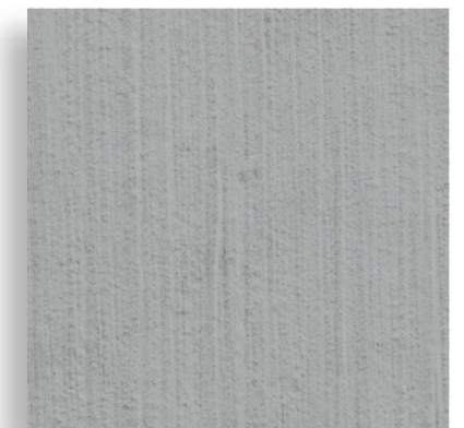
Light Broom Finished TILT-UP CONCRETE EXAMPLE
