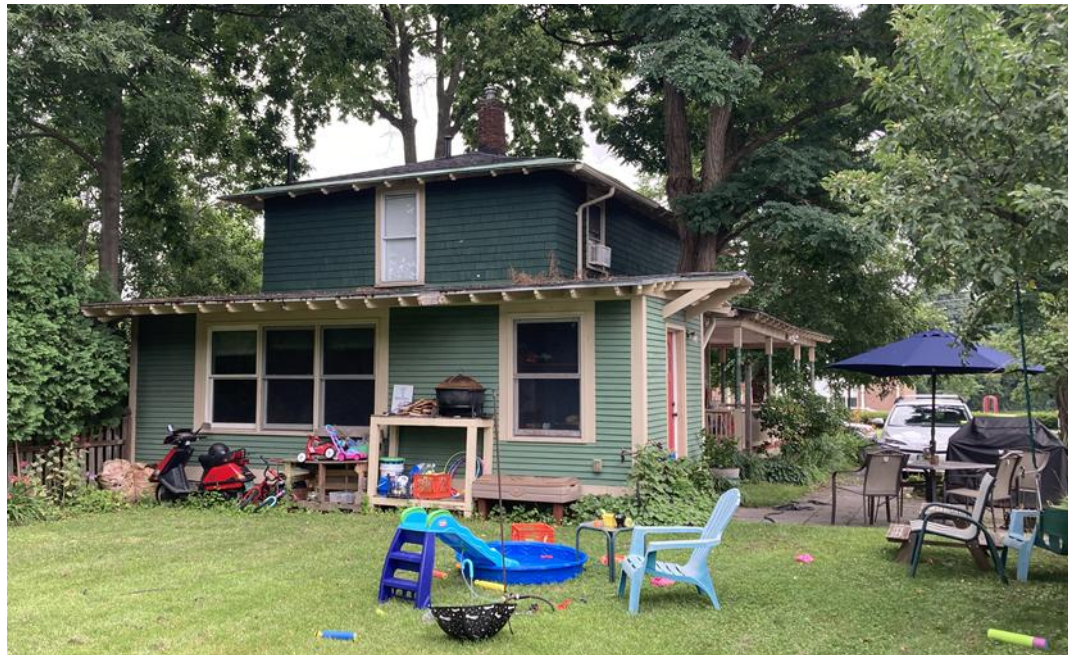
BACKYARD VIEW - AREA OF WORK
