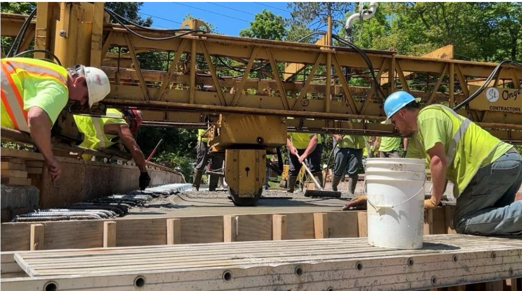
Bridge replacement over the Greenway at Rock Point
