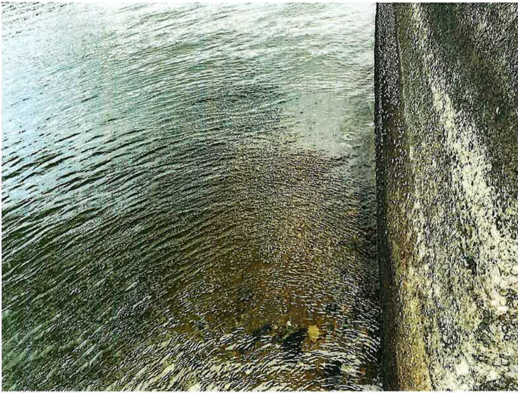
Southern Abutment – Channel Face – visible fill is fine sand.
