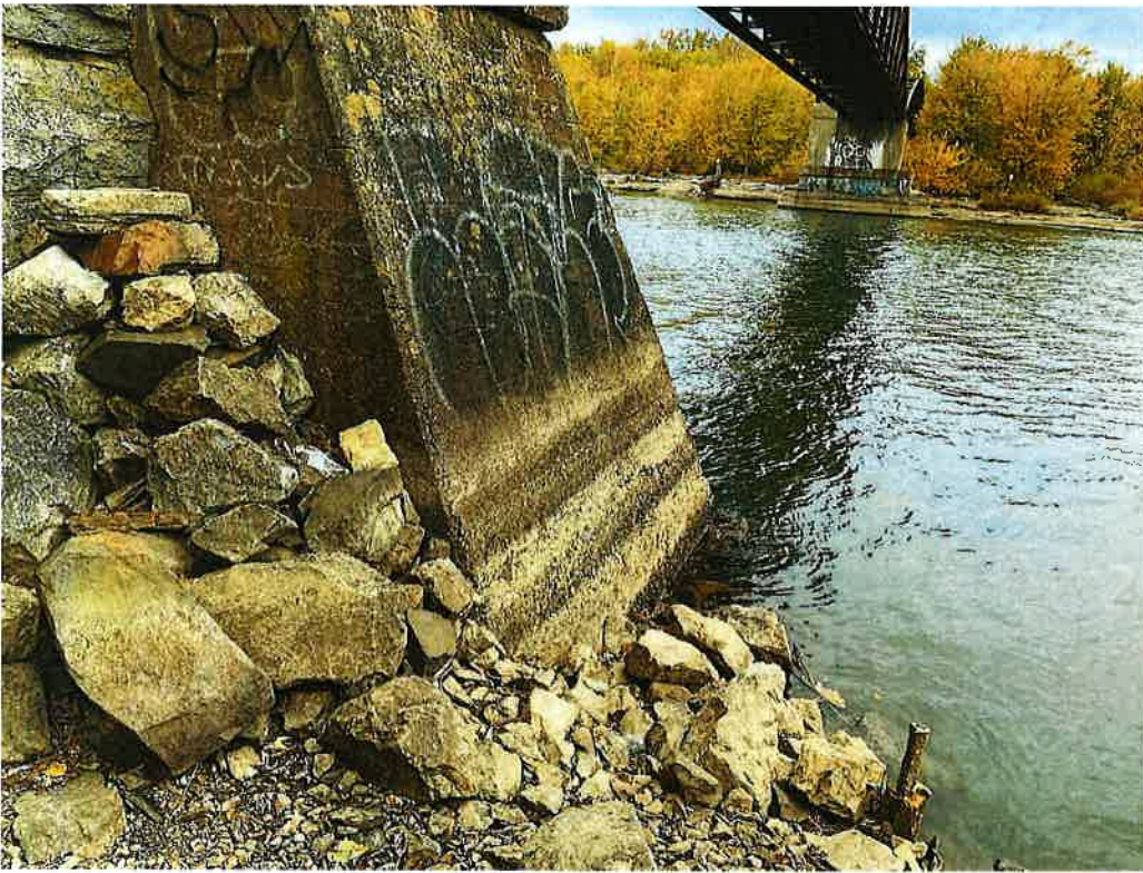
Southern Abutment – Upstream. Granular material above and below waterline. Stone is primarily 1' diameter or smaller.
