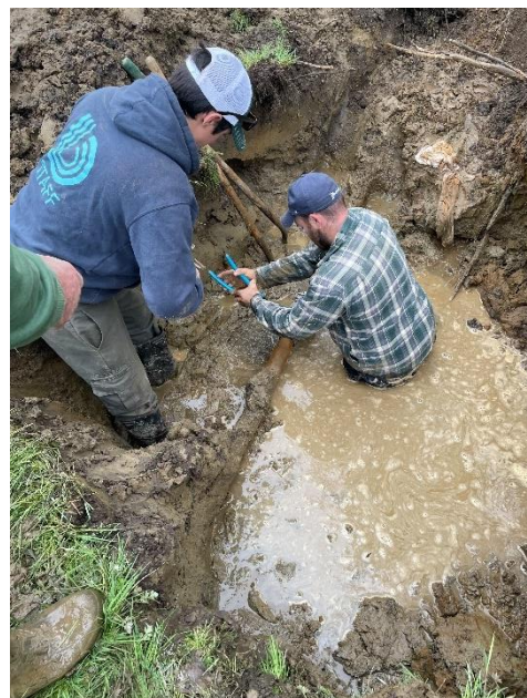
Water line repairs at North Beach
