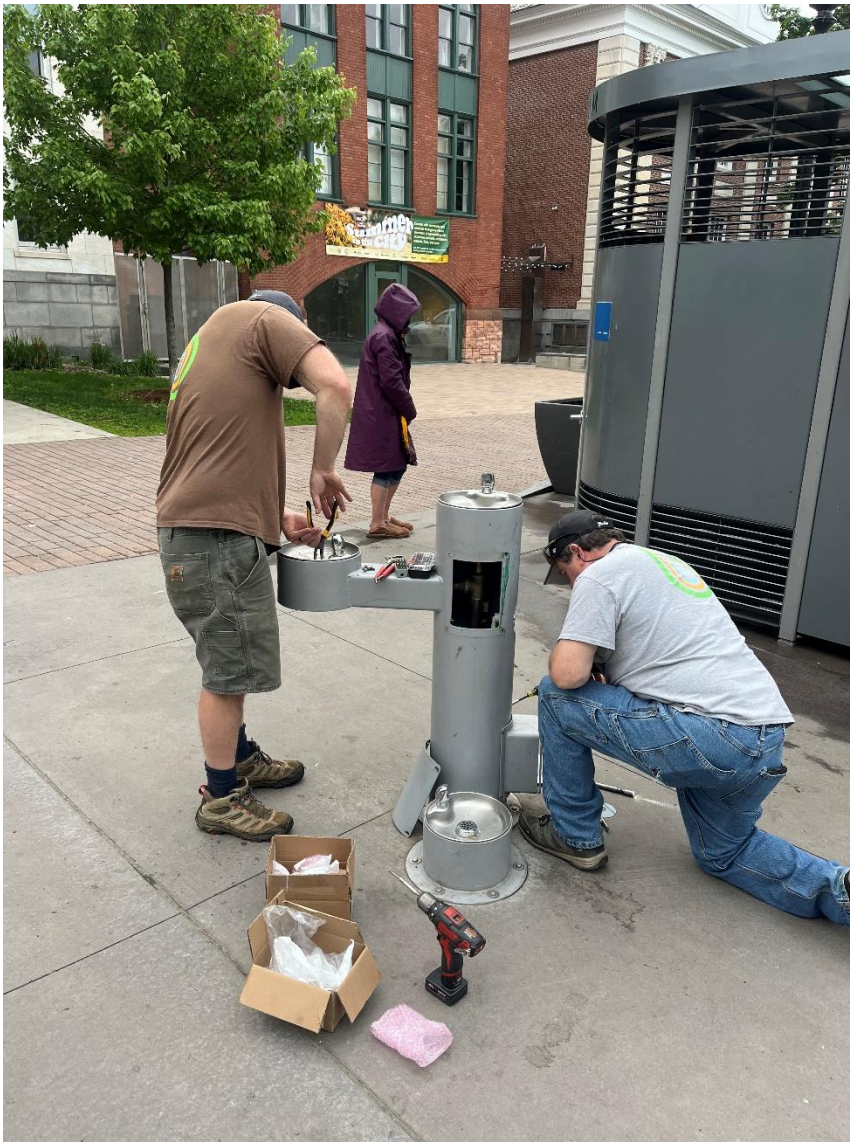
Fixing the fountain at City Hall Park
