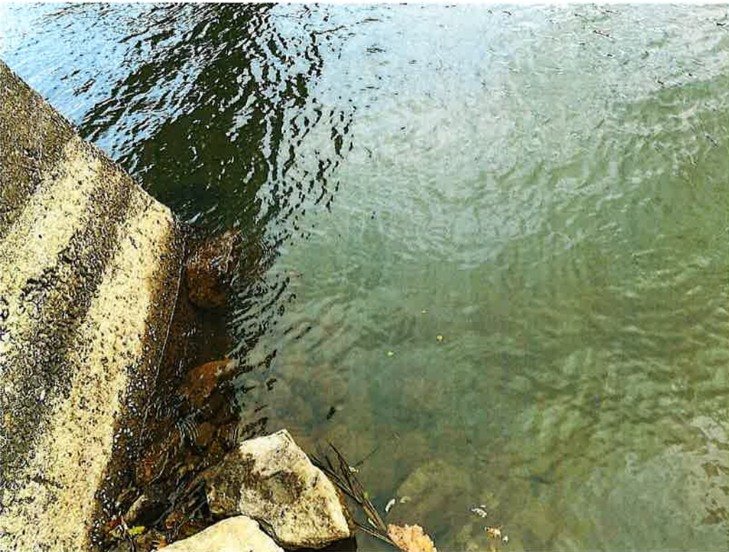
Southern Abutment – Upstream. Granular material above and below waterline. Stone is primarily 1' diameter or smaller.
