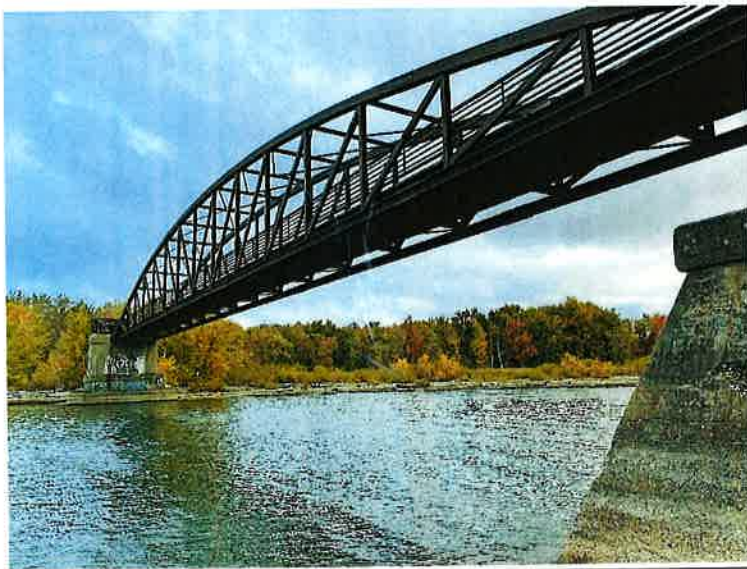
Bridge from southern abutment looking north.
