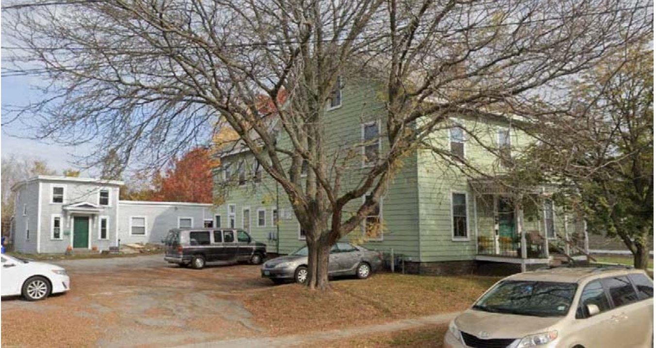
PRE-FIRE VIEW FROM SOUTHWEST
