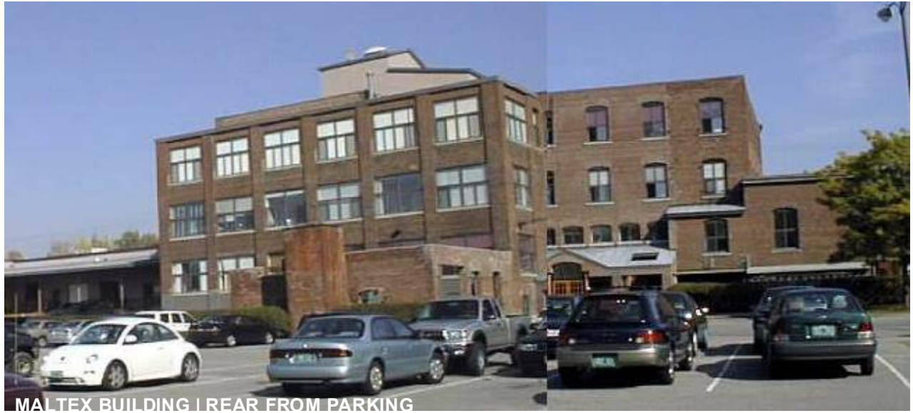
MALTEX BUILDING | REAR FROM PARKING
