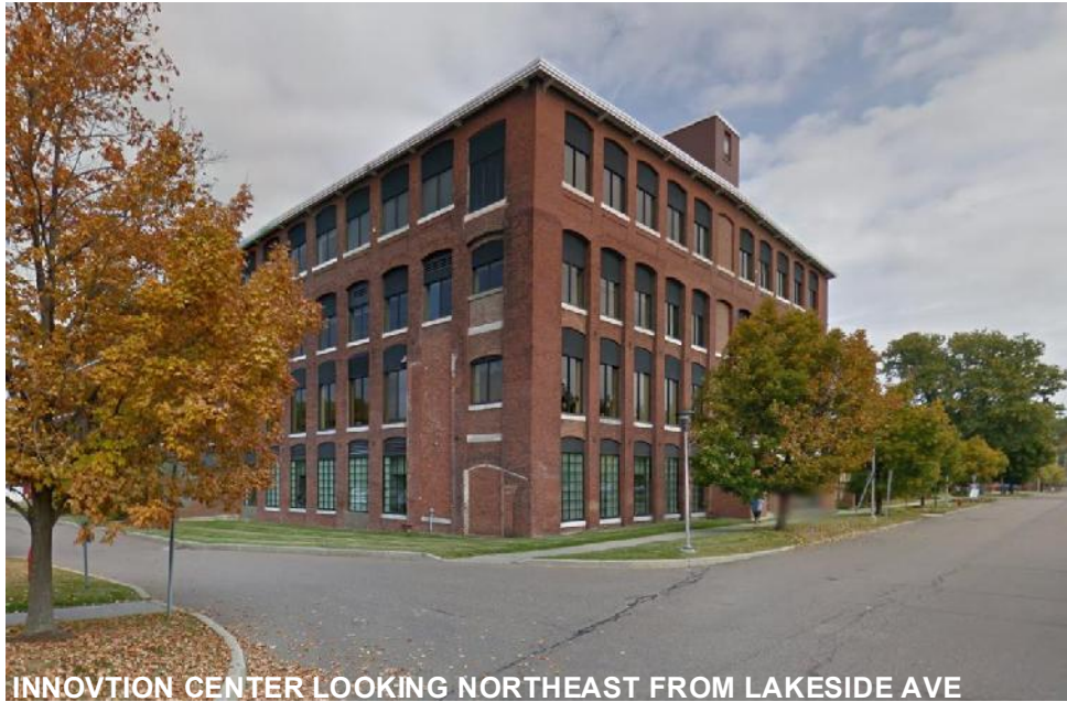
INNOVATION CENTER LOOKING NORTHEAST FROM LAKESIDE AVE
