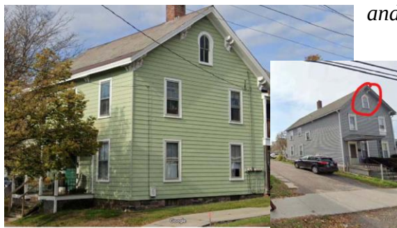
PRE-FIRE VIEW FROM SOUTHEAST
