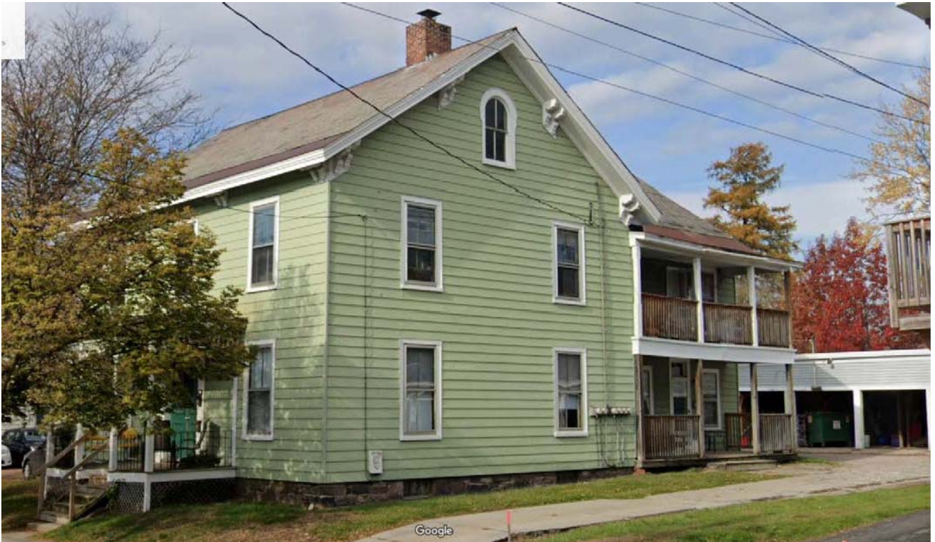
PRE-FIRE VIEW FROM SOUTHEAST
