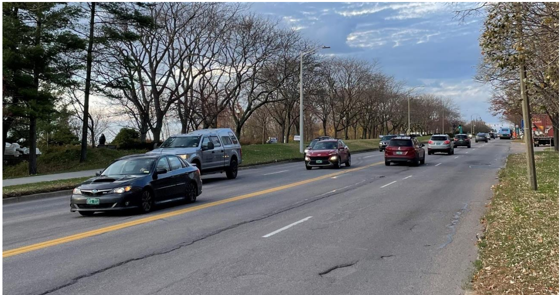
Figure 16 Four-Lane Cross-Section between College and Cherry Street
