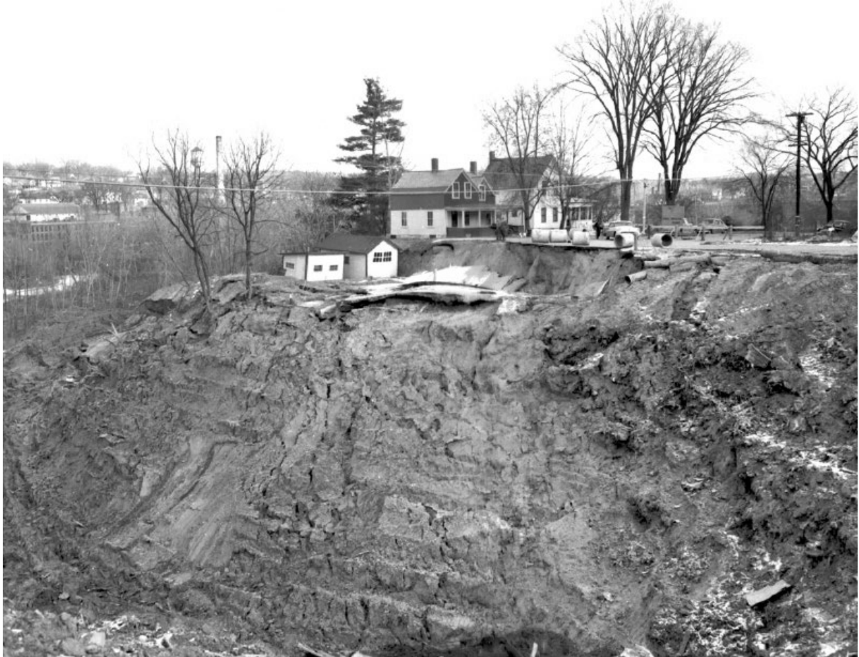
Photograph 1: View looking at the slope failure in November, 1955 which displaced large volumes of non-native fill material. Knight Consulting Engineers, Inc. in 1984 and Bennett and Bierman in 2024 cited the potential cause for this slide as excavation for a stormwater culvert installation. Photograph courtesy of the University of Vermont's Silver Special Collections Library.
