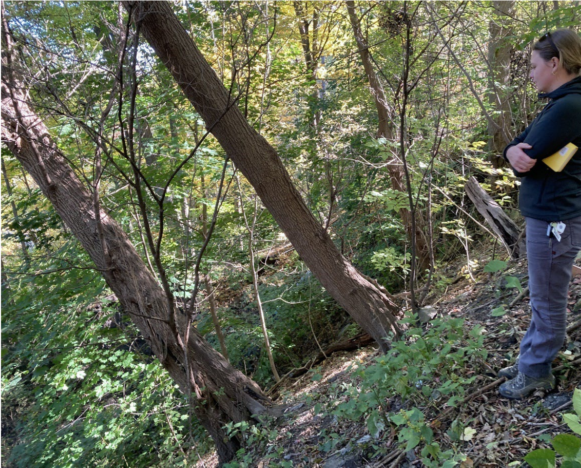
Photograph 5: View facing east showing tree trunks leaning downslope on the Parcel. The geologist in the frame provides a reference for vertical orientation.
