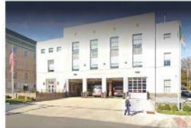
Central Fire Station
