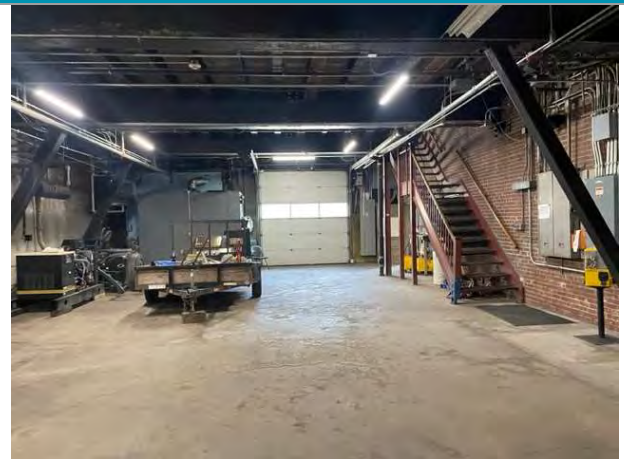
FIRE HOUSE LOWER LEVEL
