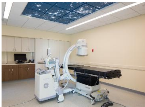
NOISE AND VIBRATION CONTROL
