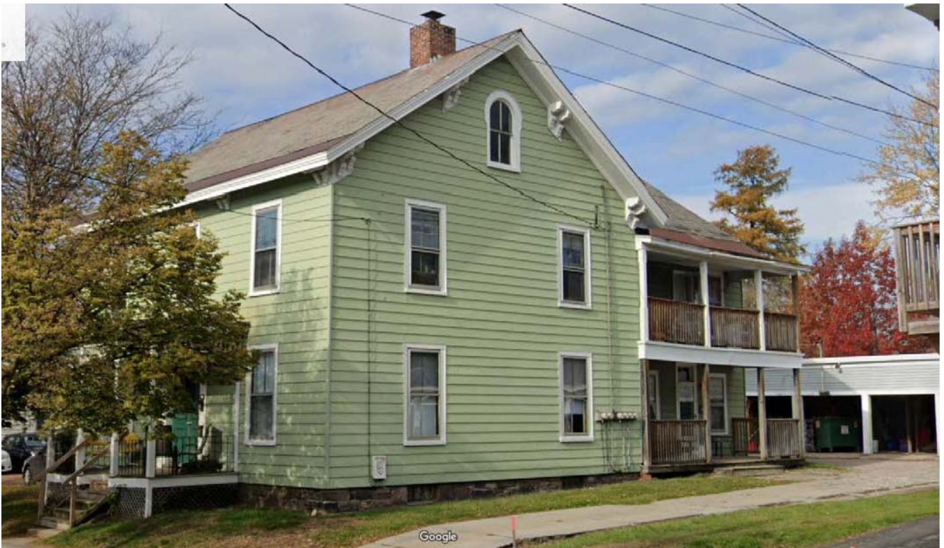
PRE-FIRE VIEW FROM SOUTHEAST
