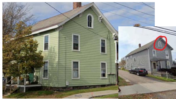
PRE-FIRE VIEW FROM SOUTHEAST
