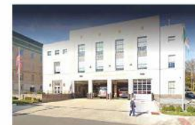
Central Fire Station
