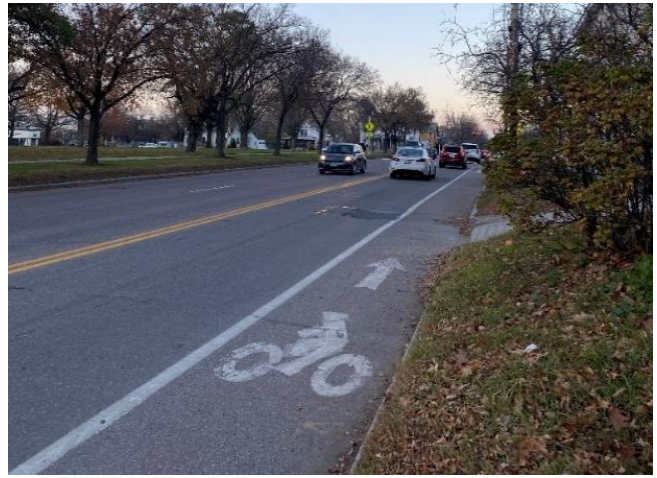
Figure 7 Bike Lane between Pearl and Sherman Street
