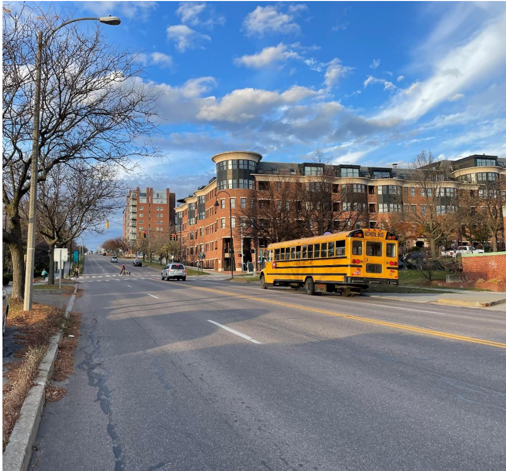
Figure 1 Battery Street Looking North Toward the College Street Intersection
