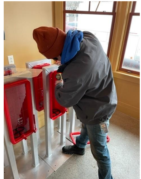
Installing fire extinguisher boxes for the frames made by Marina Manager, Rob Peterson
