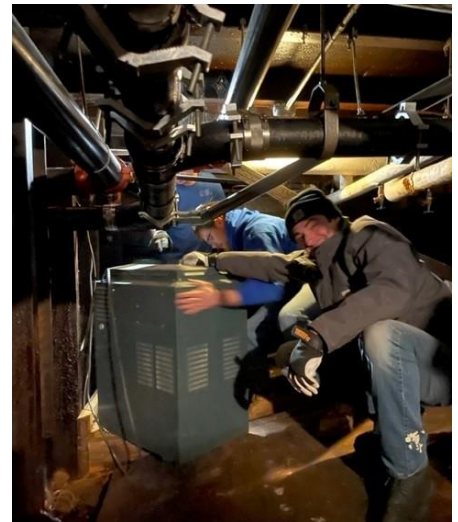
Removing the boiler under the Boathouse – cramped quarters!
