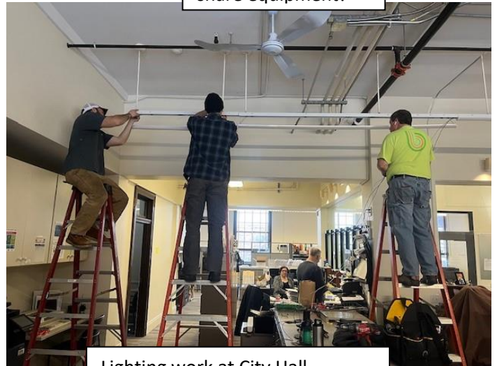
Lighting work at City Hall
