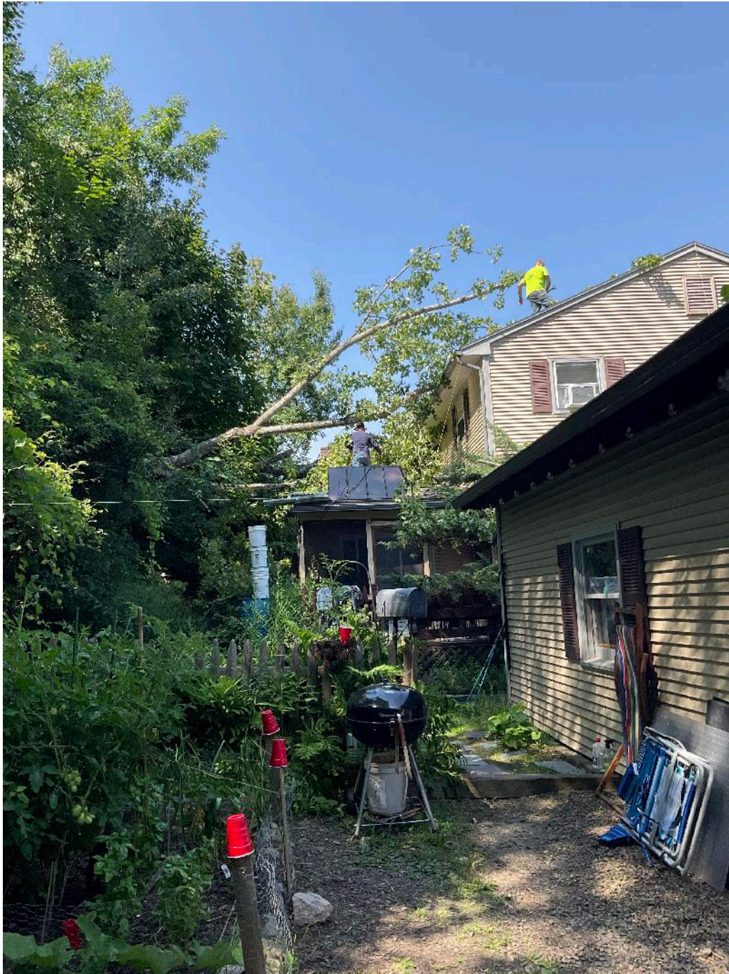
Photo 1: Green Mt. Habitat for Humanity contracted "excavator" Ray Piche and unidentified worker trespassing on the roof of our home (Rockland Condomiums, 3 Rockland St.), hurriedly attempting to remove the tree they felled onto it. July 22, 24, approximately 2:30PM
