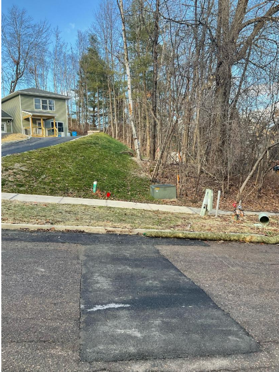
Photo 9: Retaining hill constructed along property line during August, September, October by Green Mt. Habitat for Humanity. Natural grade visible to the right; constructed, steep grade on the left. Photo taken 12/31/24
