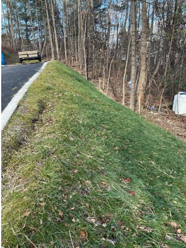
Photo 10: Retaining hill constructed by Green Mt. Habitat for Humanity. Natural grade visible to the right; constructed, steep grade to the left. Photo taken 12/31/24
