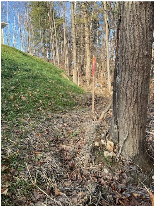
Photo 10: Retaining hill constructed by Green Mt. Habitat for Humanity. Natural grade visible to the right; constructed, steep grade to the left. Photo taken 12/31/24
