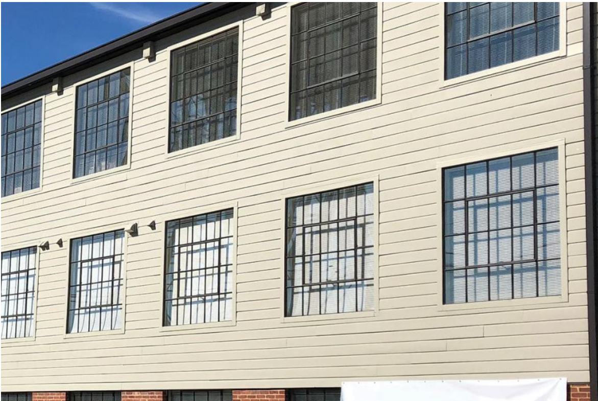
Figure 21. A mineral polymer composite siding was available in the profile very similar to the historic siding. The replacement siding was used where the original material was almost completely missing beneath a more modern covering. Areas where the original wood was largely intact were replaced with matching wood to sustain more of the material integrity of the building. Photo: Belk Architecture.
