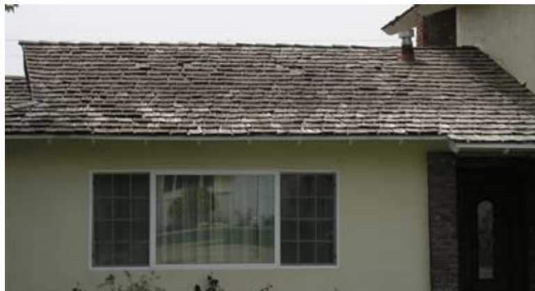
Figure 1—Cedar shake roof.
