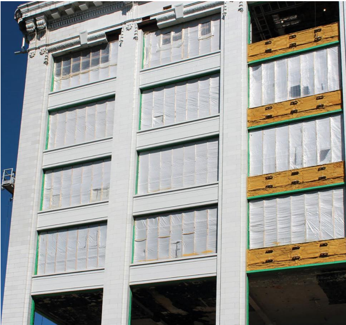
Figure 18. Missing historic terra cotta spandrel panels on all floor levels were recreated utilizing glass fiber reinforced concrete (GFRC) replacements. New spandrels were fabricated as individual components and attached with metal clips between historic terra cotta piers. Photo: Kris Frail, Dewberry.
