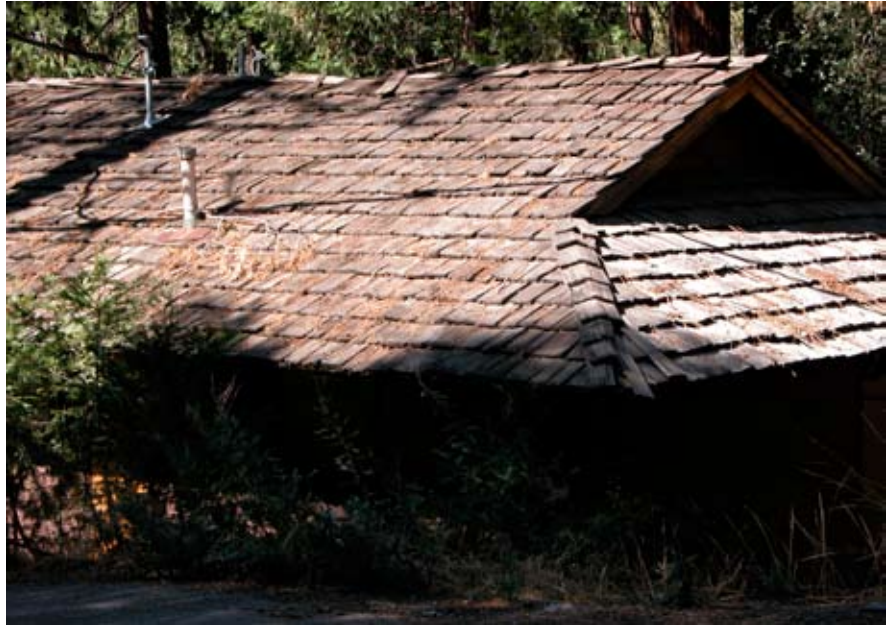
Figure 2—Cedar shake roof.
