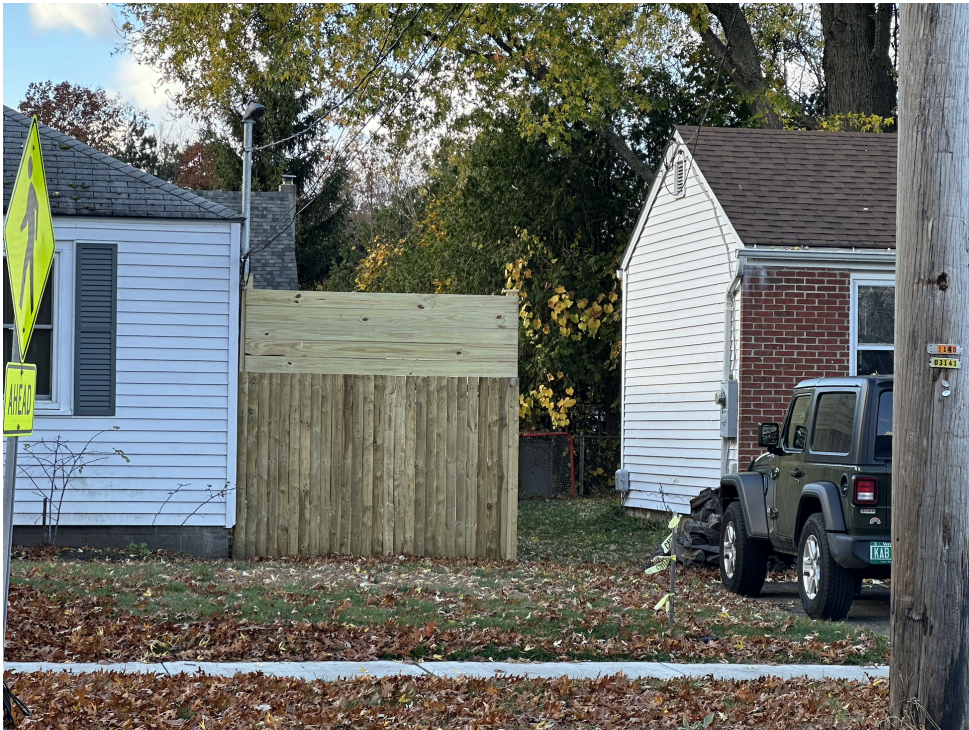
Appendix B. Photo showing the excessive height and nonconformity of the 8' foot fence.
