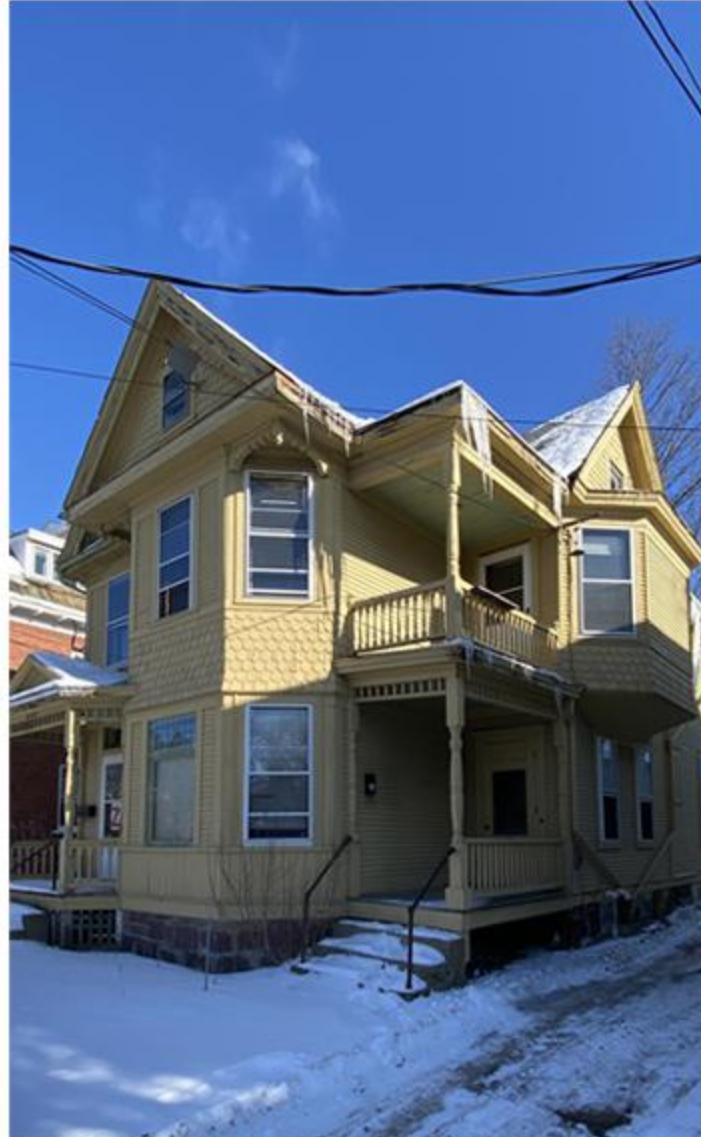
FROM HOUSE DRIVEWAY
