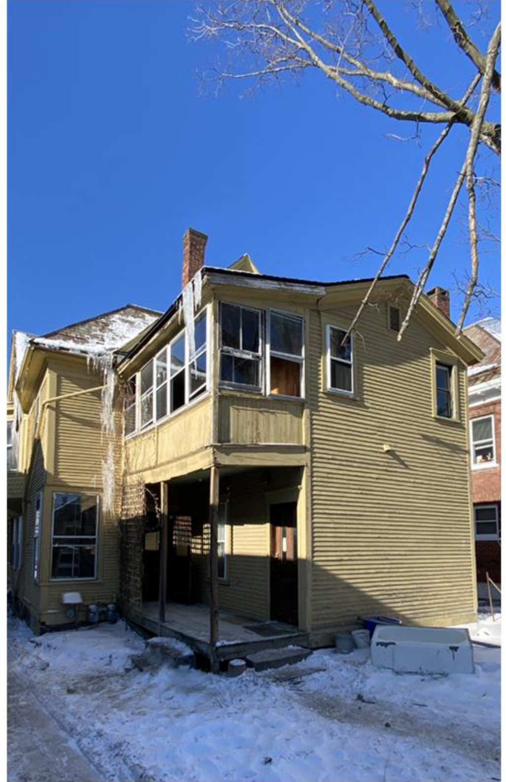
REAR OF BUILDING - FROM PARKING AREA
