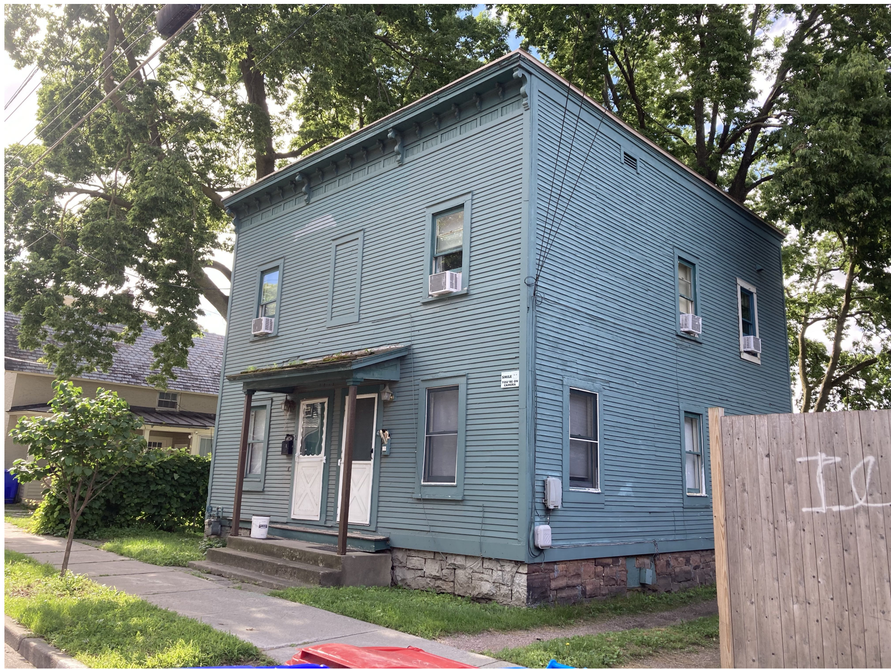
SIMILAR BUILDING STYLE IN NEIGHBORHOOD
