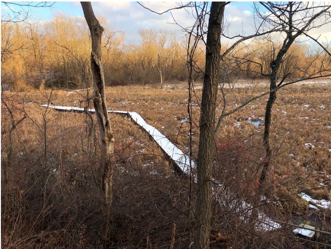
View of Wetlands Walk North Boardwalk from the stairs on the western approach showing expanse of boardwalk through the wetlands. Photo taken December 13, 2023.
