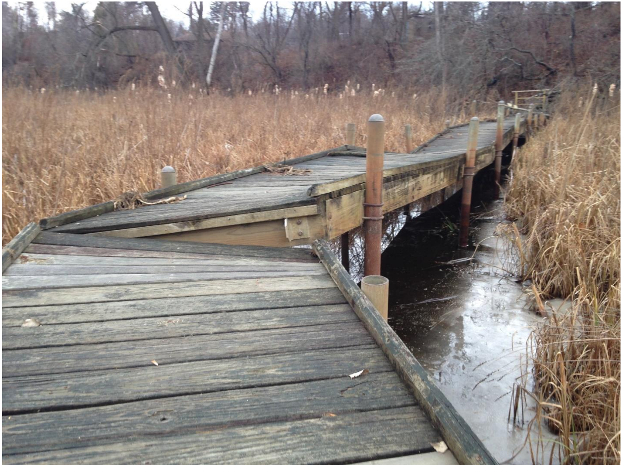
Dislodged sections of board looking west (above). Broked steel anchor support (below). Photos taken December 10, 2019.
