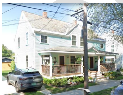
59-61 Central Avenue Reconstructed chimneys
