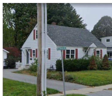
1999 North Avenue Chimney removal possible
