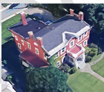
342 Pearl Street Repair/repointing 5 chimneys
