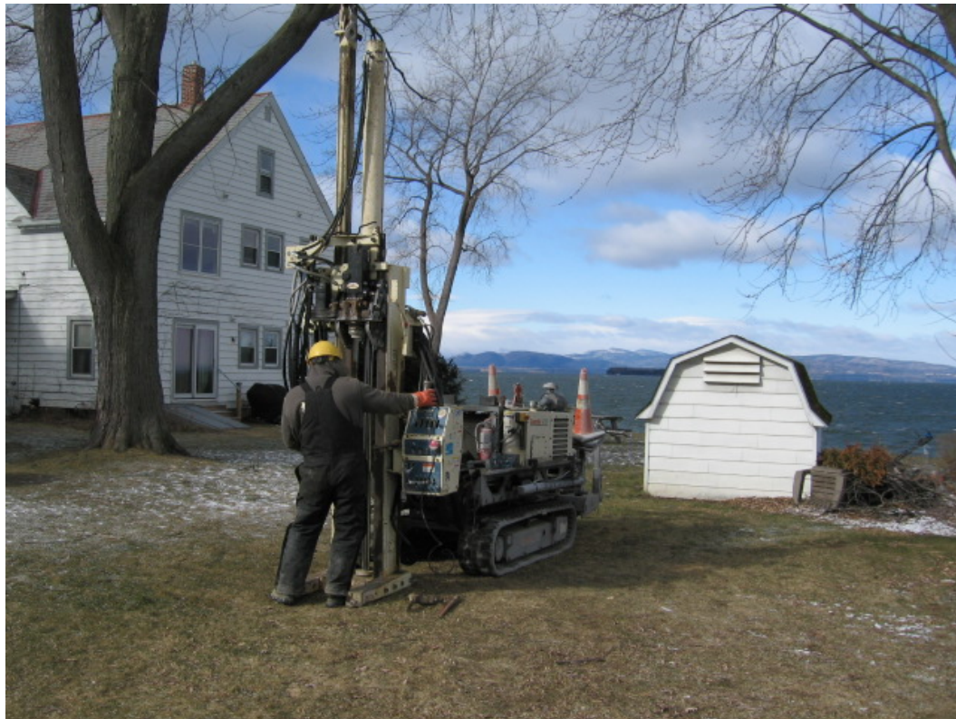
view of boring location
