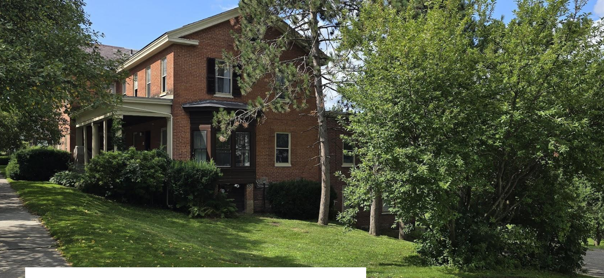
Existing Building – NE Corner
