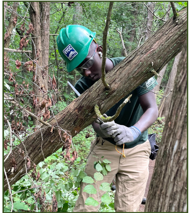
Aiden of Session 2 Burlington Crew saws through a log for the turnpike structure at Arms Forest.
