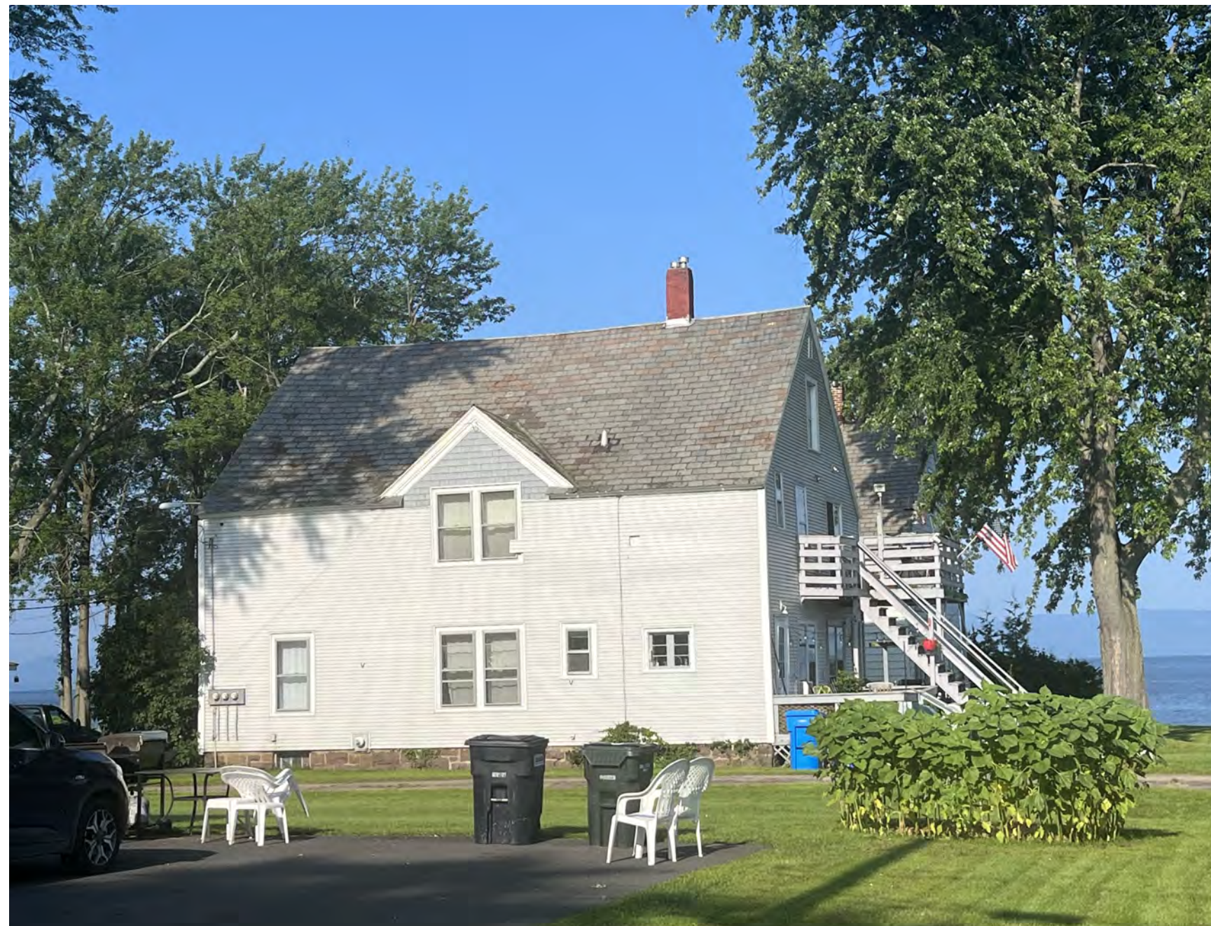
EXISTING BUILDING EAST ELEVATION
