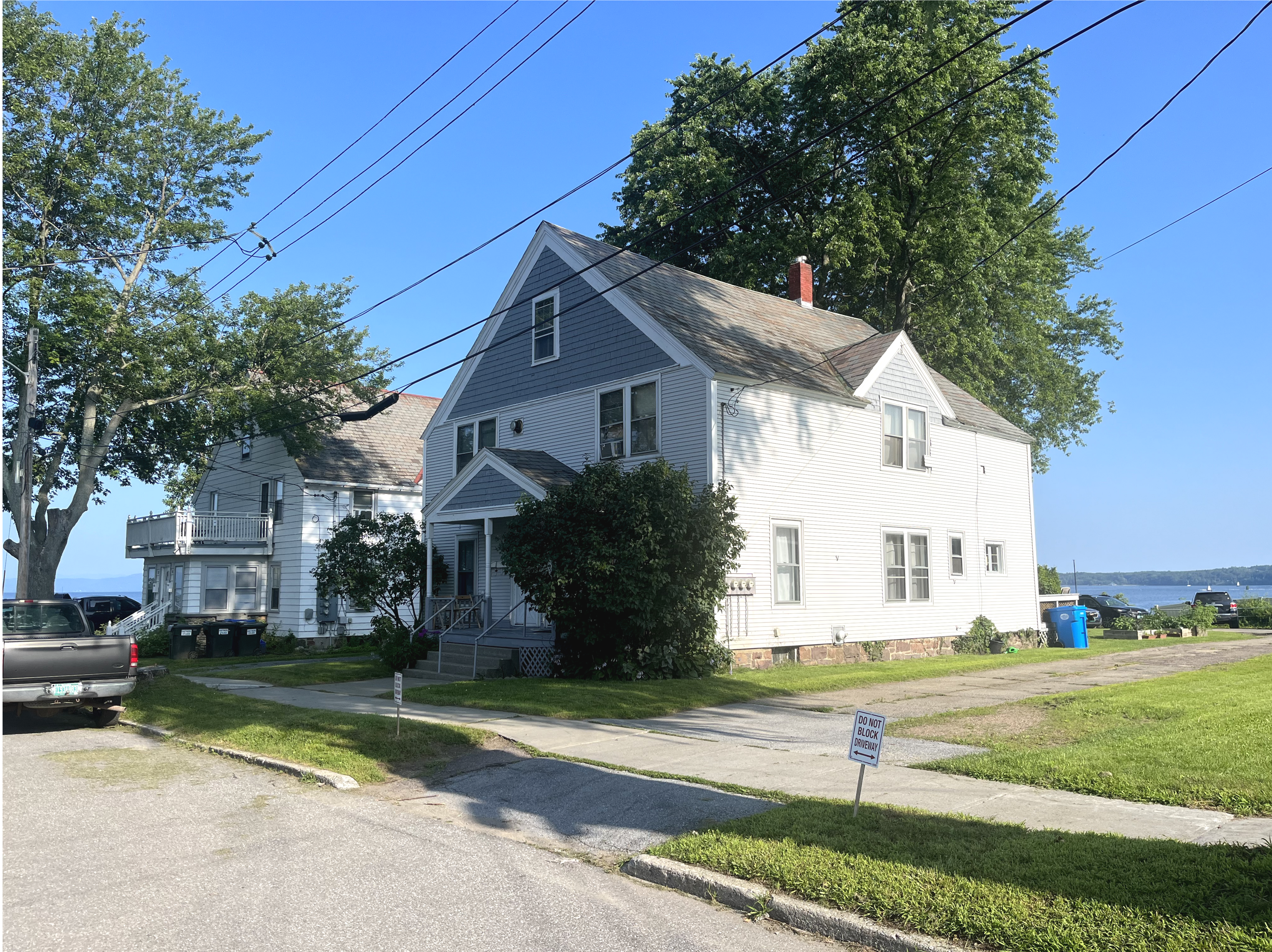
EXISTING BUILDING VIEW FROM SOUTH EAST
