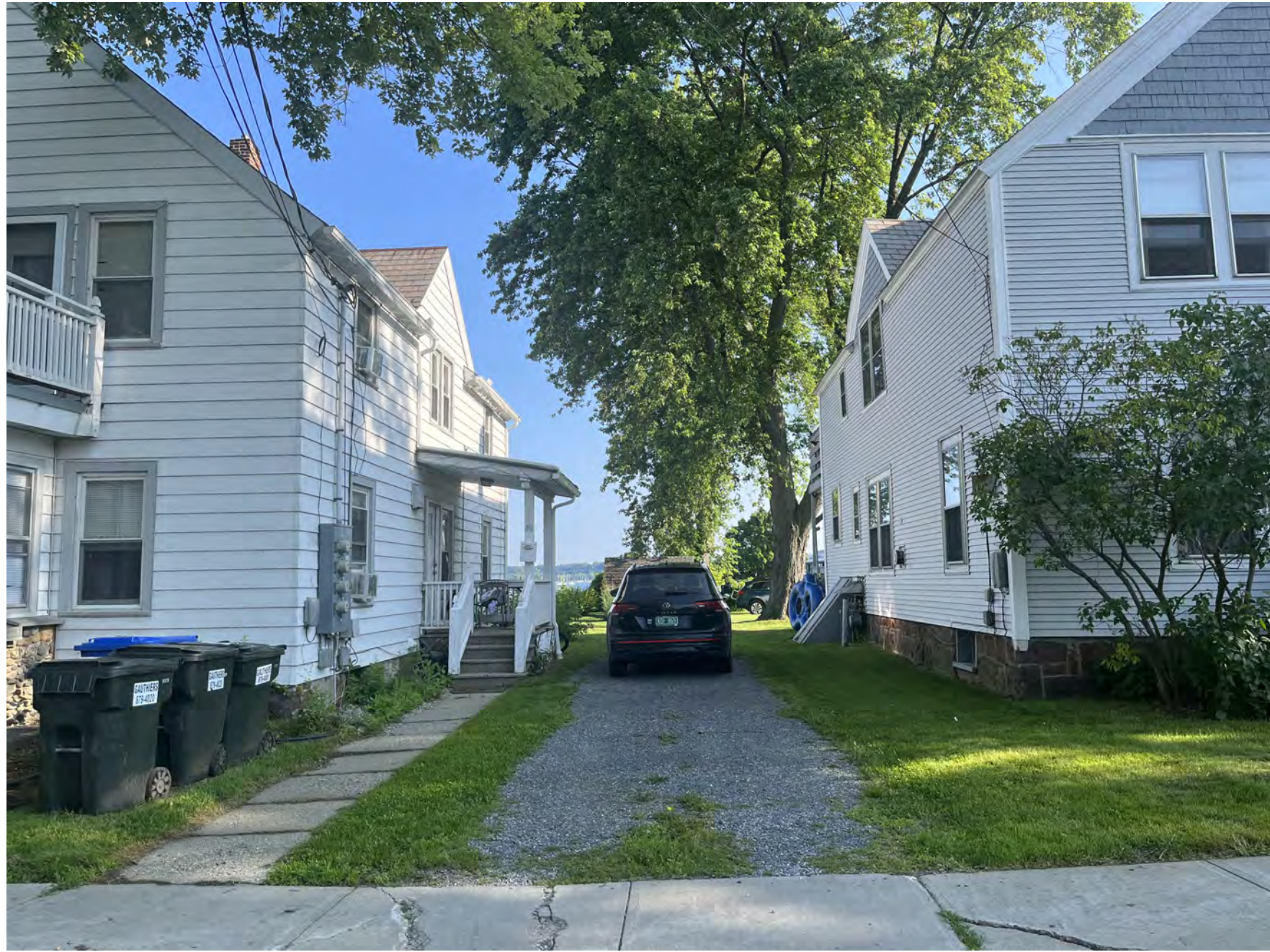
EXISTING BUILDING WEST ELEVATION (RIGHT) • STREET VIEW.
