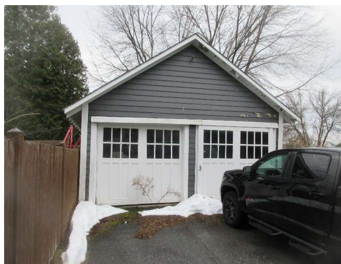
PHOTO 2: Garage looking south
