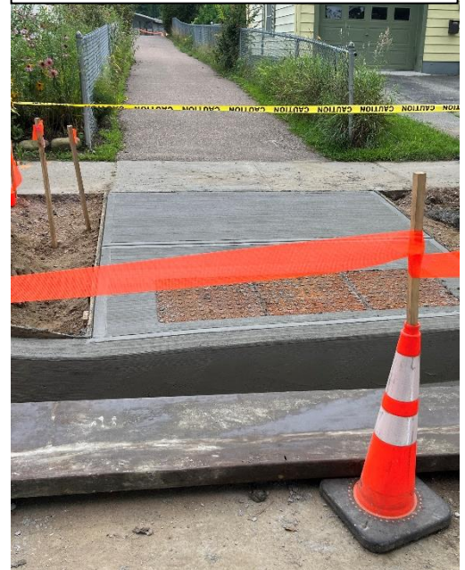
New accessible entrance to James Ave easement
