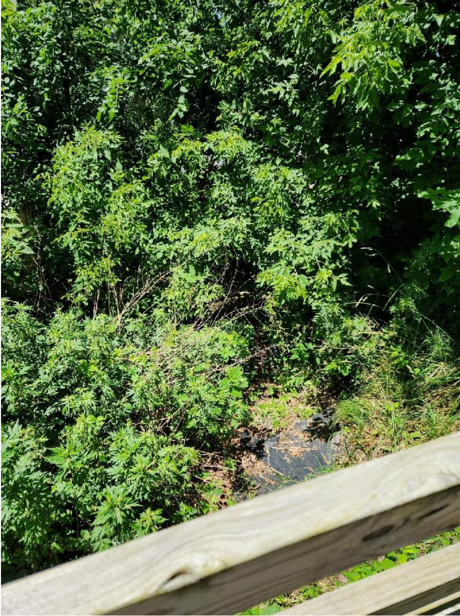
Existing culvert outlet
