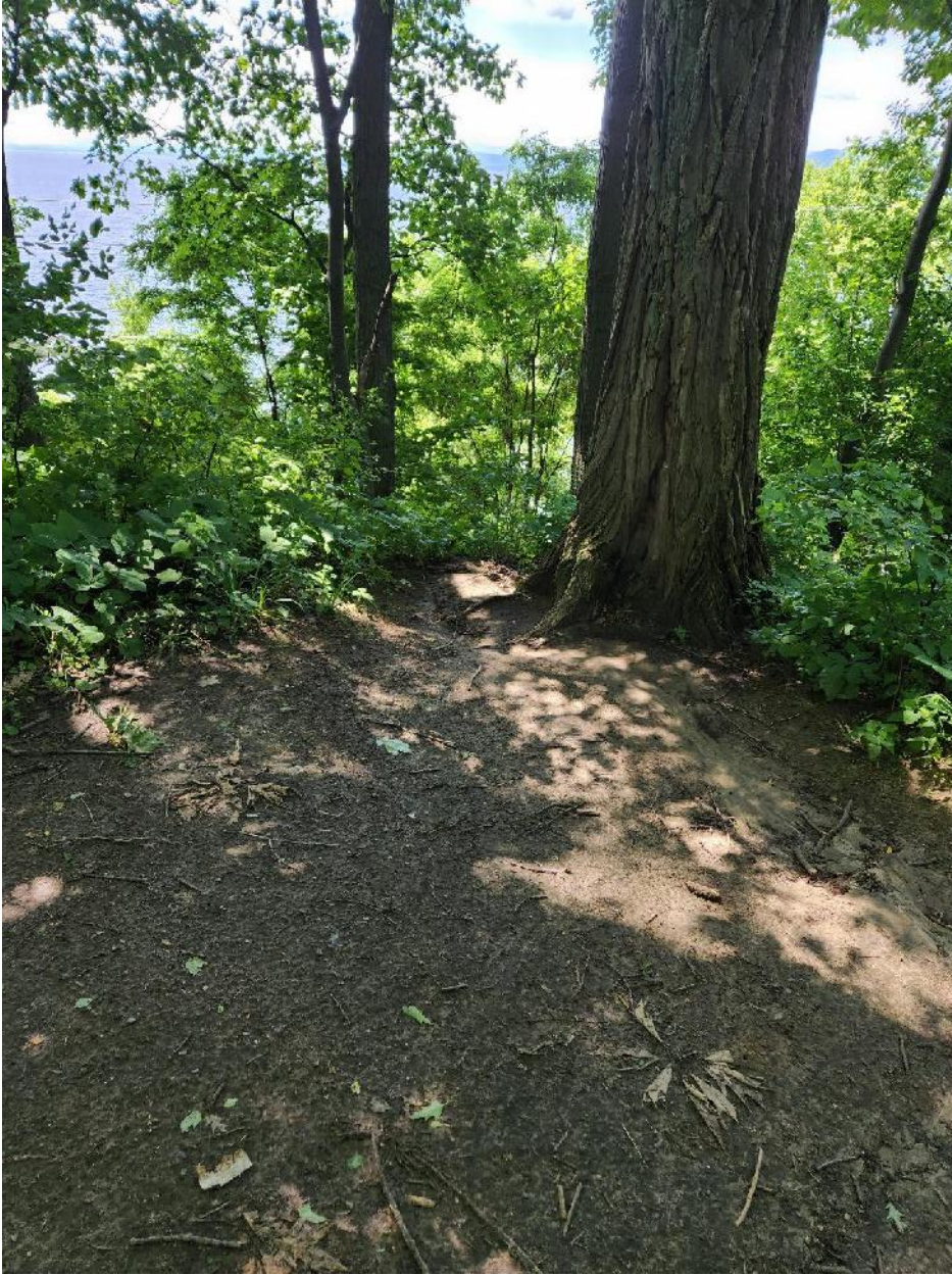
Eroding area at top of hill
