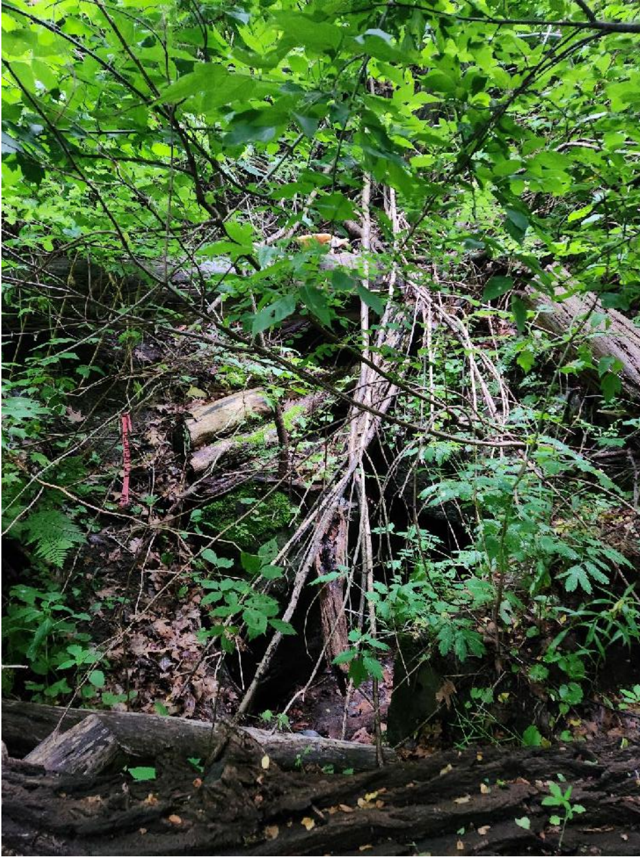
Uphill opening of existing culvert.
