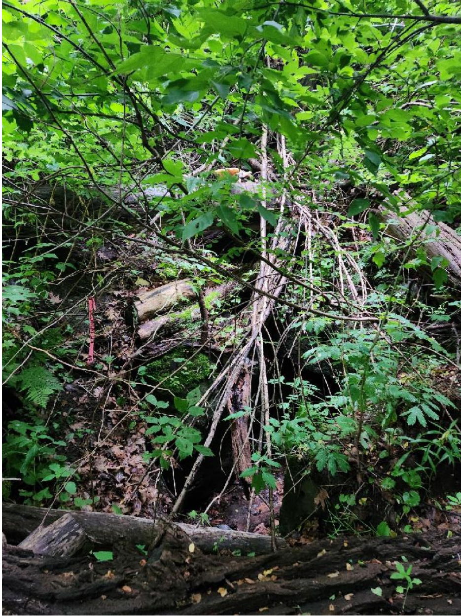
Uphill opening of existing culvert.
