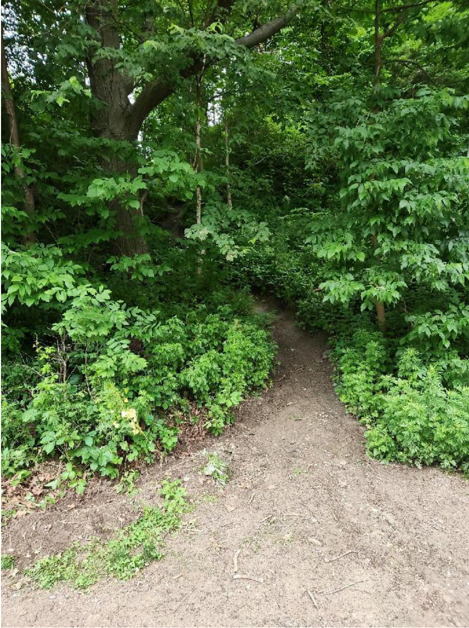
Erosion of existing path
