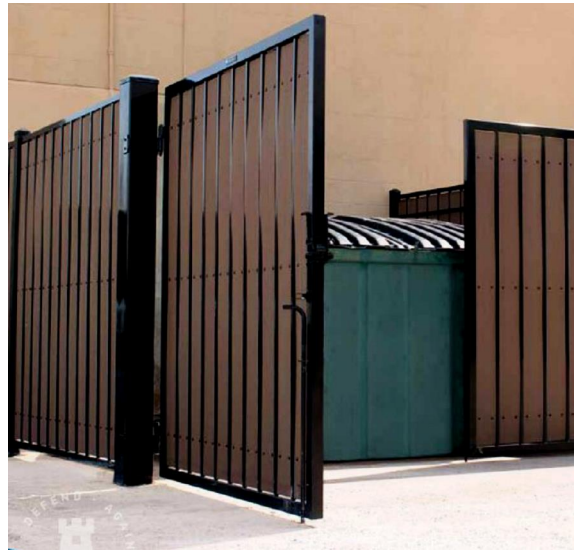
5'-0" HIGH DUMPSTER FENCING
