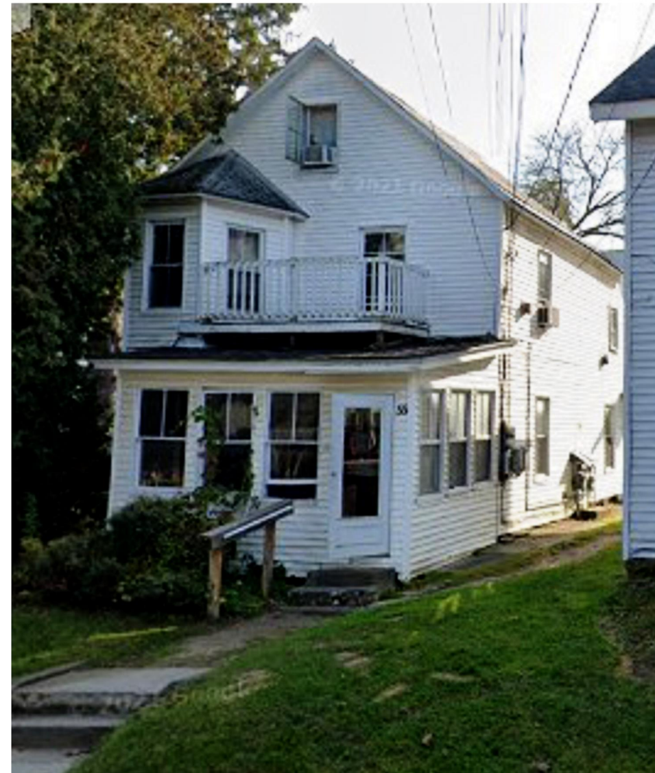
FRONT (NORTH) VIEW OF 55 CHASE STREET
