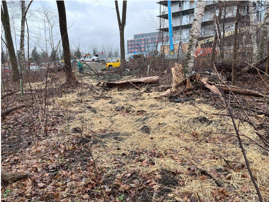
Figure 3. In some cases, the bases of trees (called “root wads”) were apparently excavated from the ground, a highly unusual practice that causes considerable soil damage.
