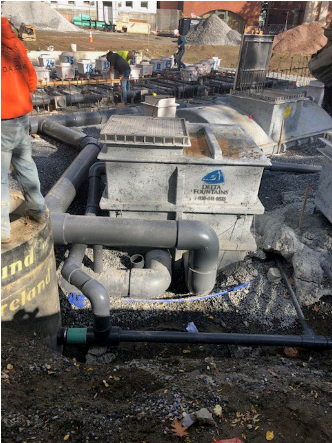
Connection to SMH #1
