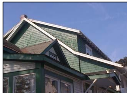
Roof with multiple pitch configurations
