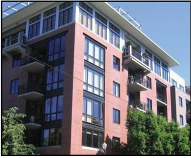
Parapet wall with projecting cornice
