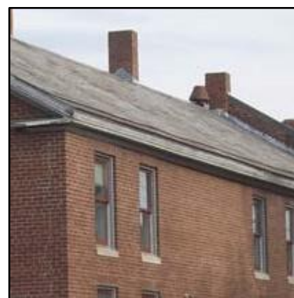
Pitched roof with enclosed eaves
