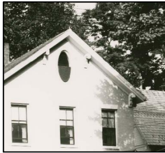
Pitched roof gable end with brackets
