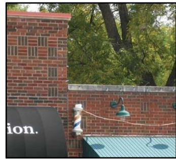
Parapet wall with coping
