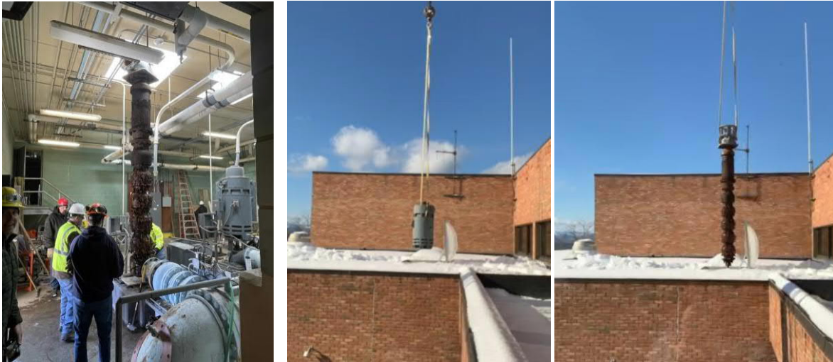
Pictures of pump motor and pump getting removed from Water Plant
