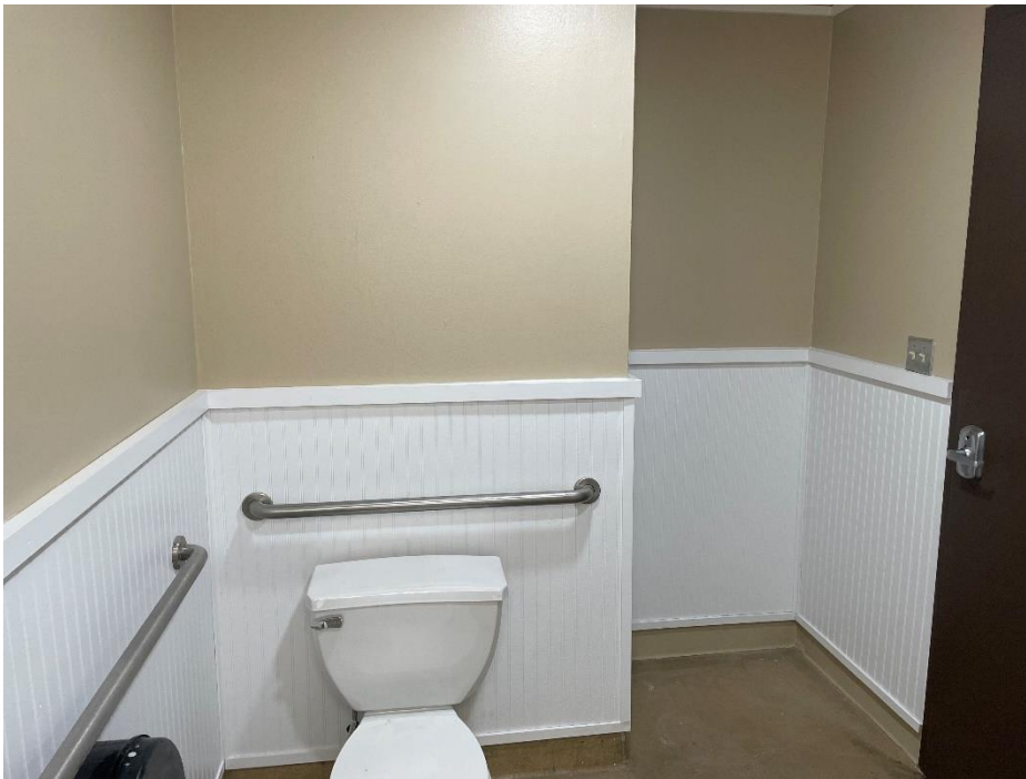
The renovation of the Perkins Pier bathrooms came out great!
