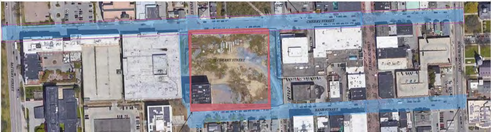
Figure 1. Image of Burlington showing the location of the project area encompassing Cherry Street, Bank Street and connections of Pine Street and St. Paul Streets to Cherry Street.
