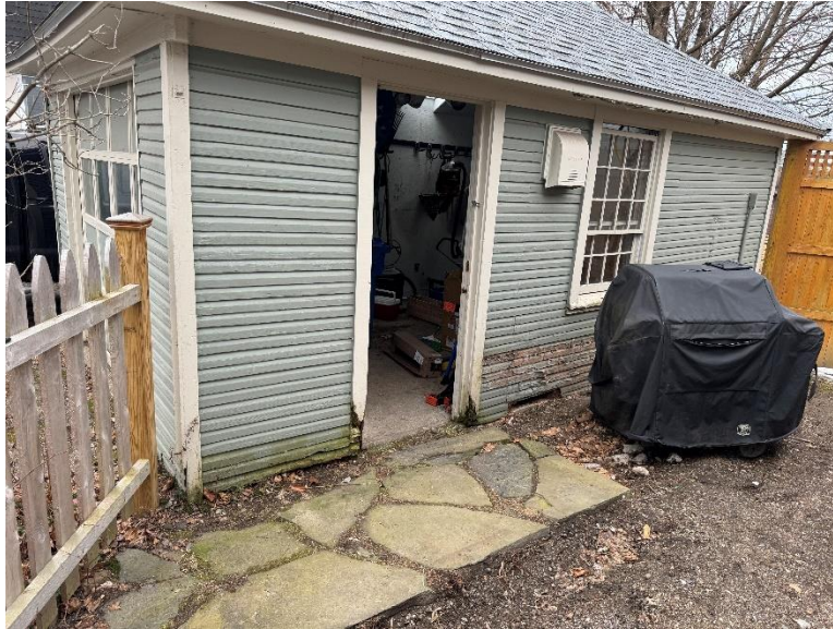
Figure 1 - Detached garage structure
