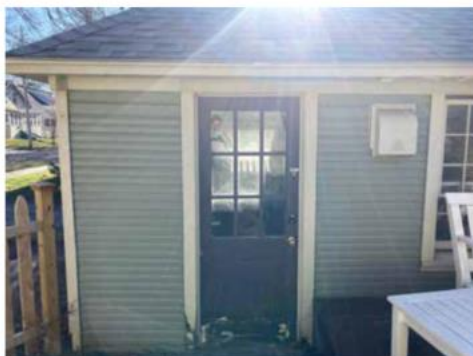
Existing garage, north facing
