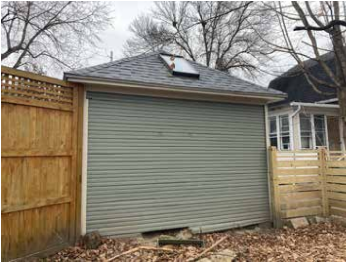
Existing garage, east facing
