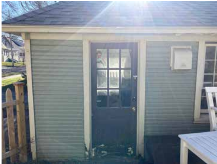
Existing garage, north facing
