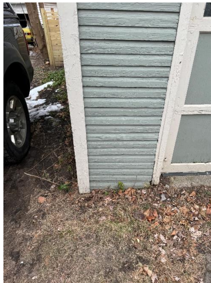
Figure 8 – South west corner of wall and wood framing below grade
