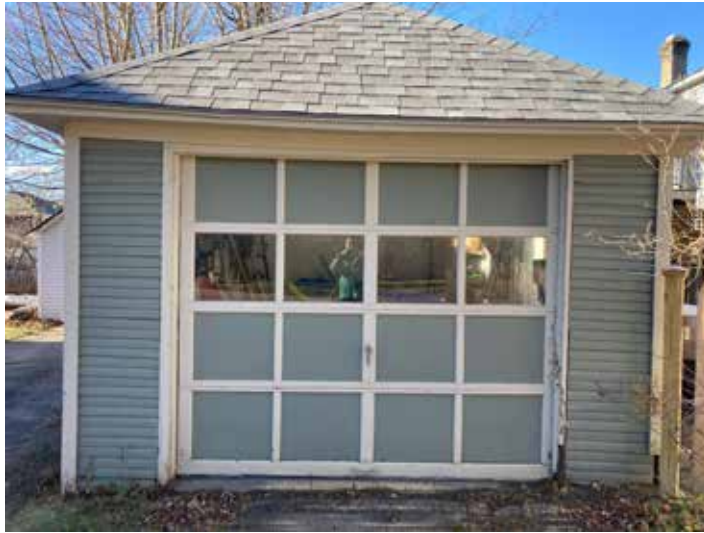
Existing garage, east facing
