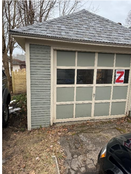
Figure 5 – East wall with garage door
