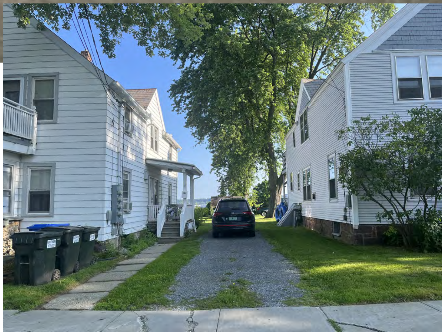
EXISTING BUILDING WEST ELEVATION (RIGHT) • STREET VIEW.
