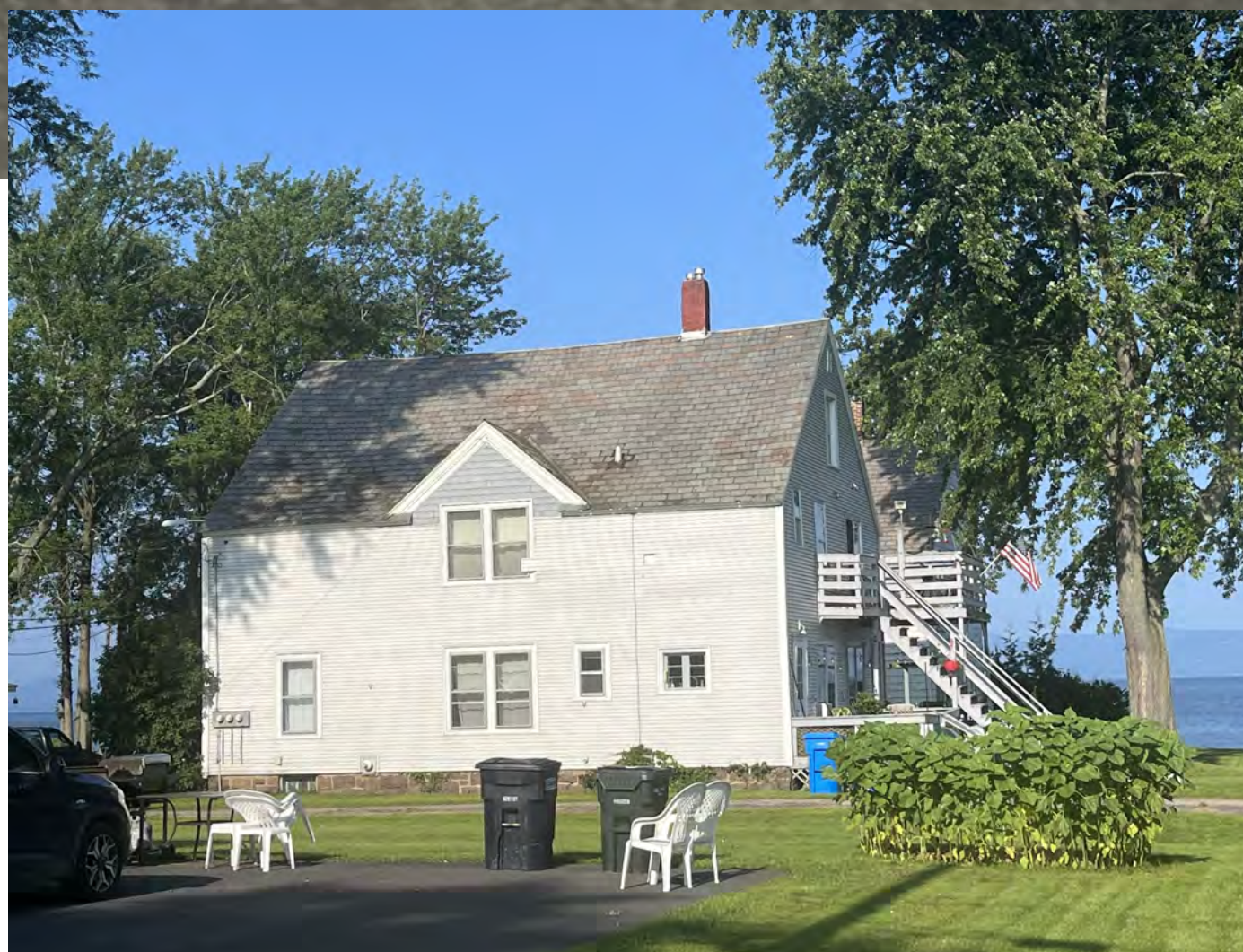
EXISTING BUILDING EAST ELEVATION
