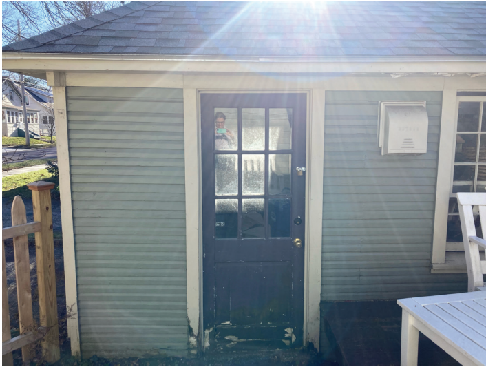
Existing garage, north facing
