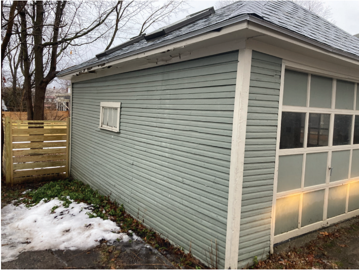
Existing garage, south facing
