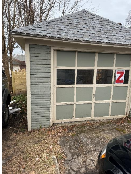
Figure 5 – East wall with garage door
