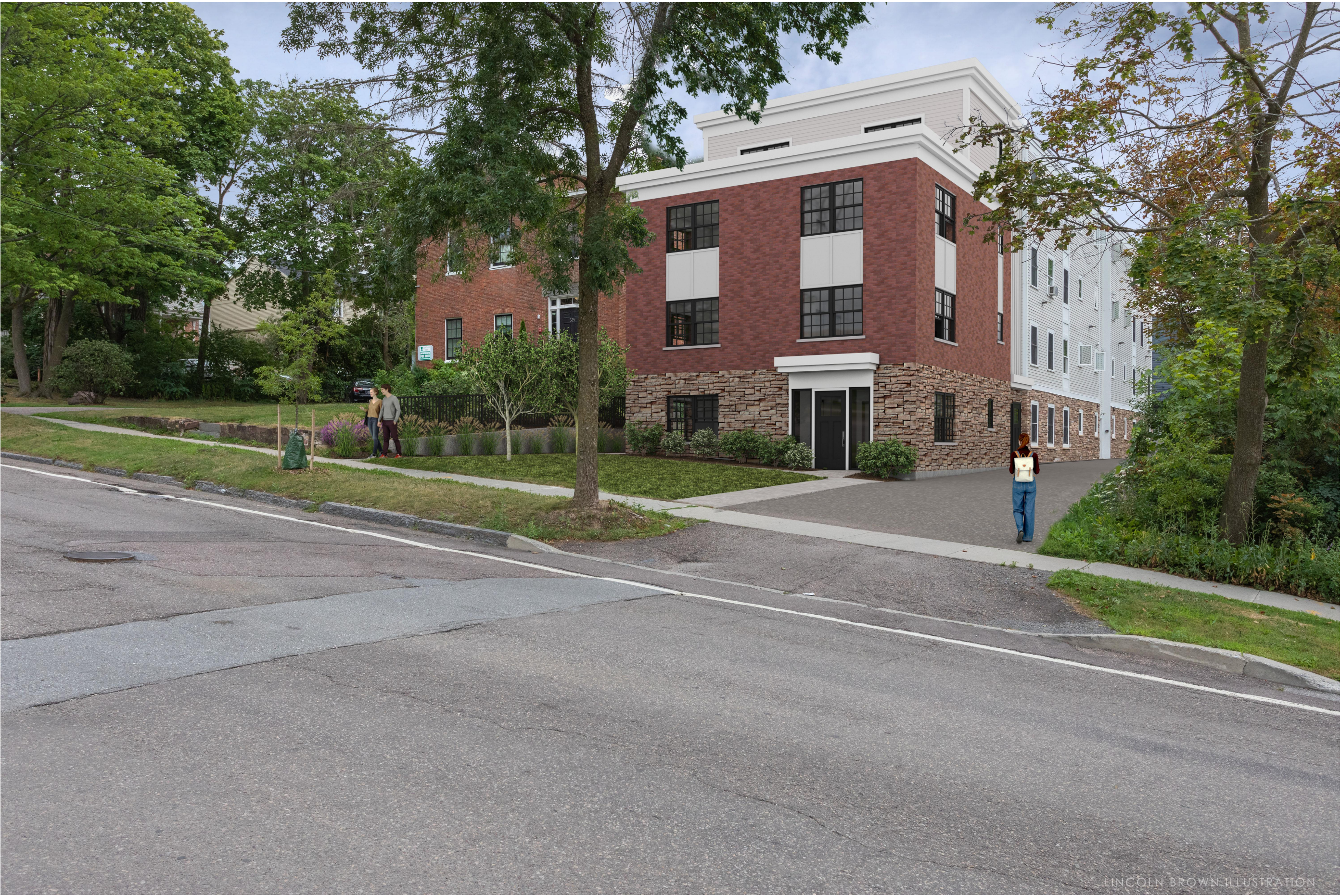
VIEW TO NORTHEAST
